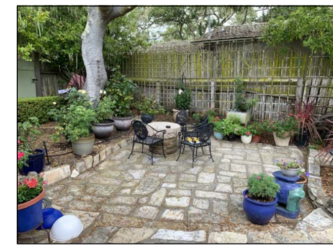
STONE PATIO UNEVEN / UNSAFE SURFACES
