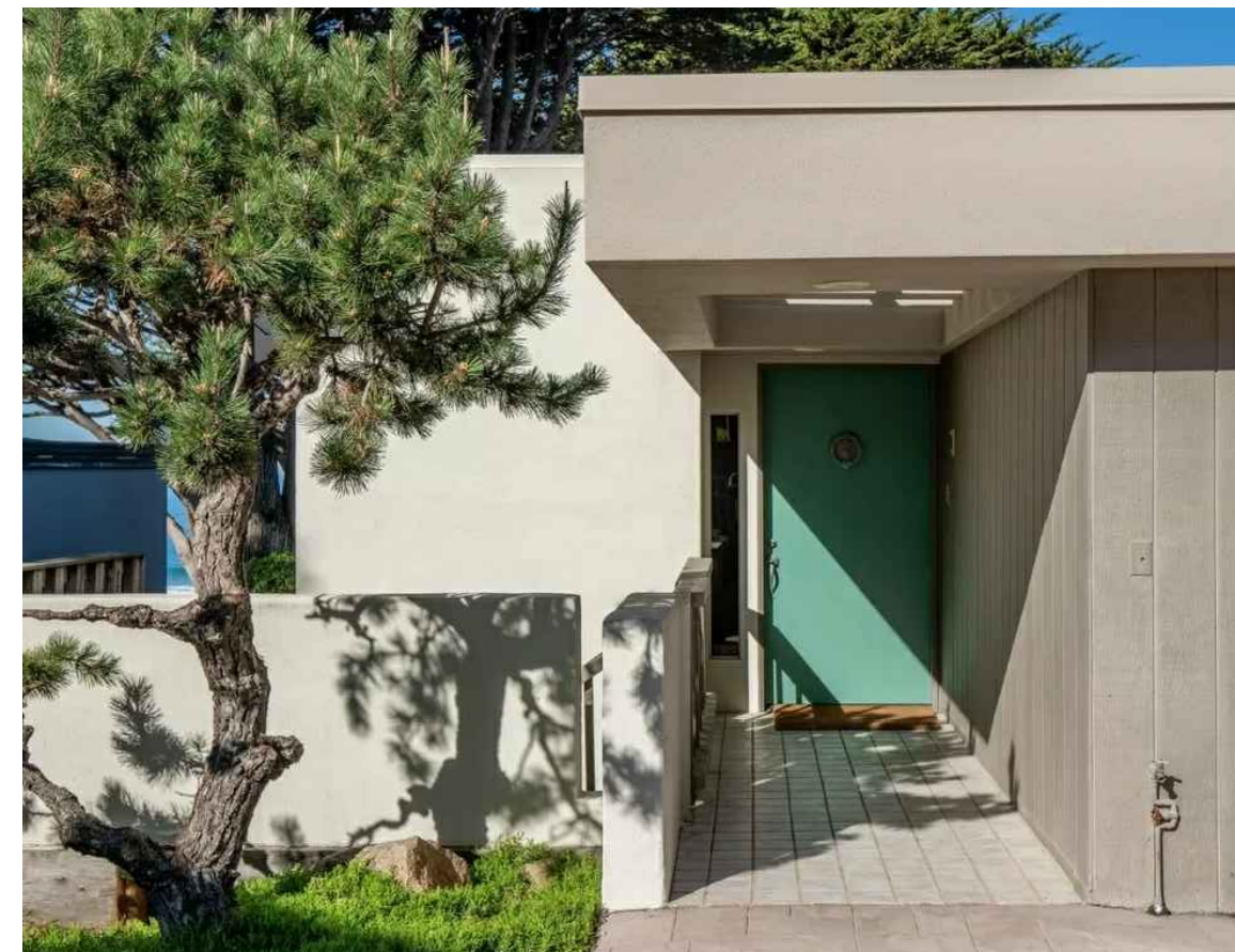
FRONT OF (E) HOUSE LOOKING WEST
