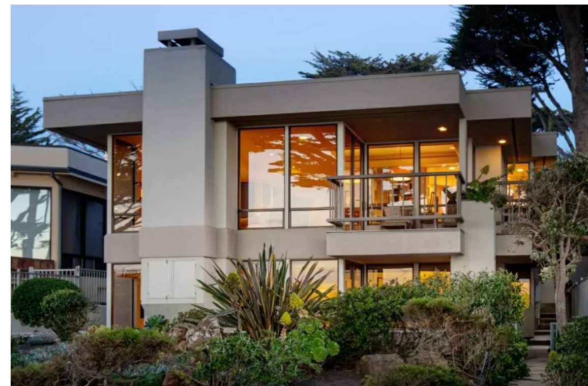
BACK OF (E) HOUSE LOOKING EAST
