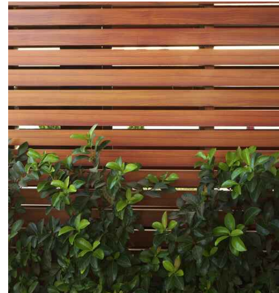
TEAK FENCE, STAINED, 1X6 BOARDS SPACED 1/2" APART
