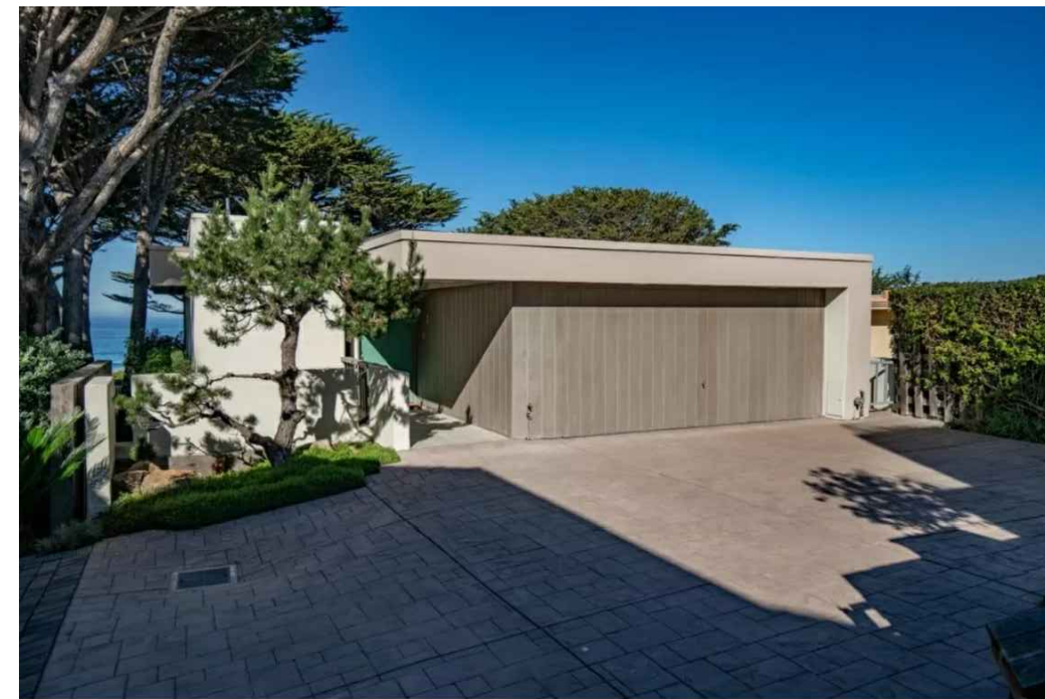
FRONT OF (E) HOUSE LOOKING WEST
