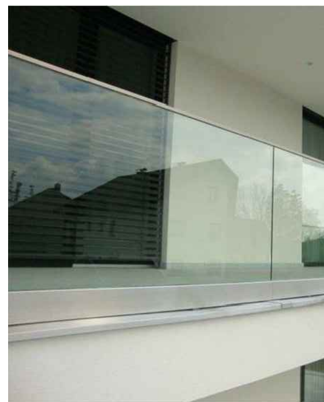
GLASS RAILING DETAIL W/ CONT. BASE
