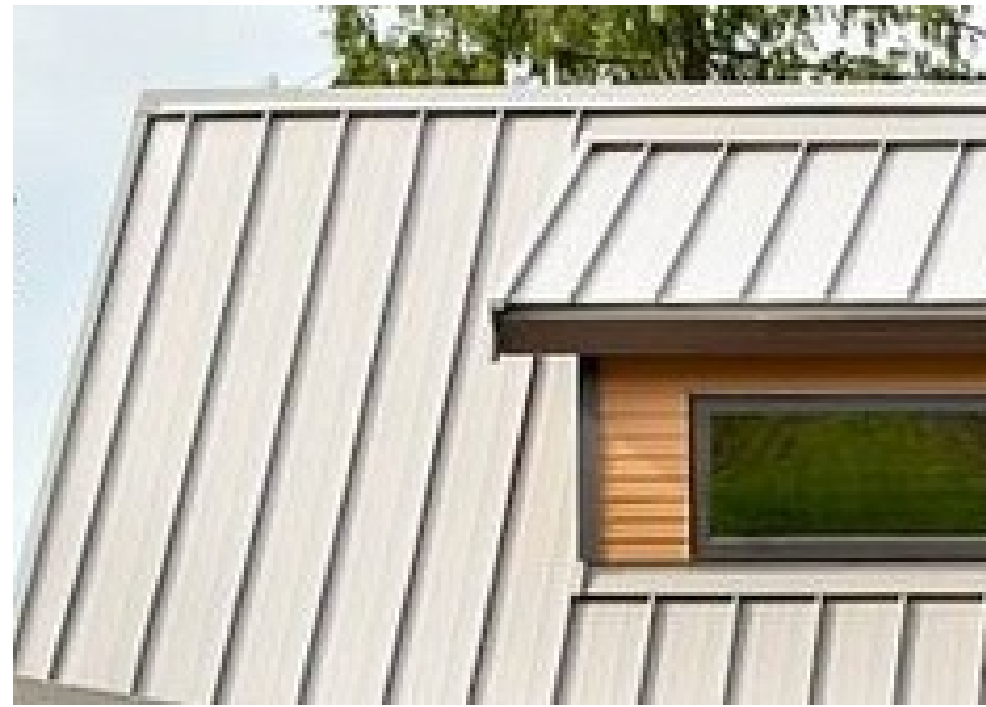
STANDING SEAM METAL ROOFING
