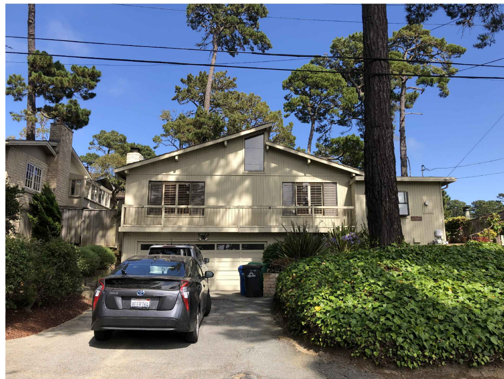
STREET VIEW OF (E) HOUSE LOOKING EAST - (E) DECK & RAILING TO REPAIR
