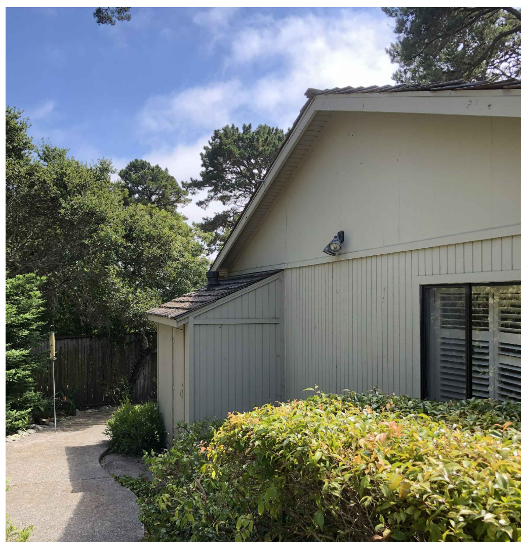
REAR OF (E) HOUSE LOOKING SOUTH - REMOVE (E) SHED & BUILD NEW 136 SF 'STUDY' ADDITION
