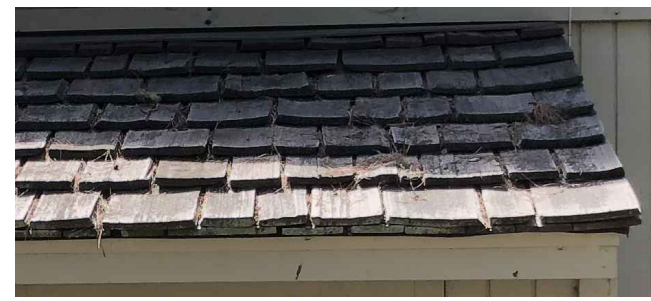
WOOD SHAKE ROOF TO MATCH (E)
