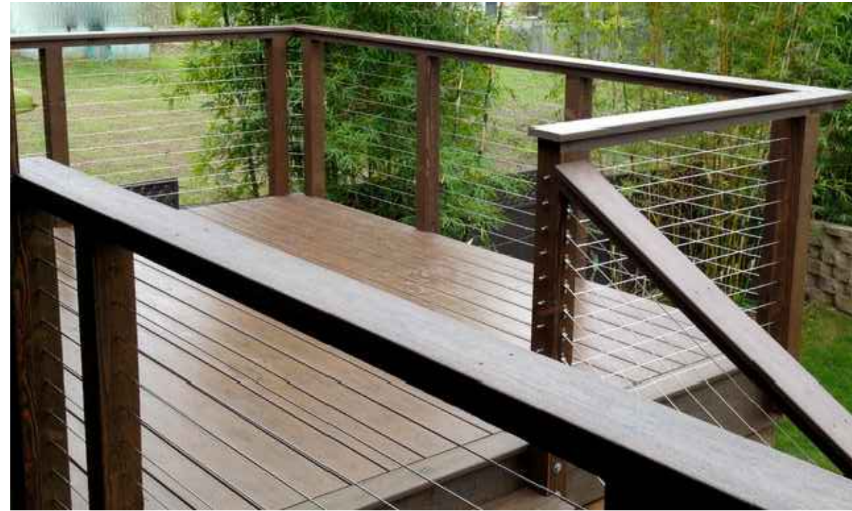
REPAIRED GUARDRAIL & DECK - KEEP (E) 4X4 POSTS, NEW 2X4 WOOD TOP RAIL & HORIZ. ALUM. CABLE RAILING
