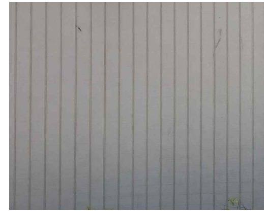
VERTICAL WOOD SIDING TO MATCH (E)
