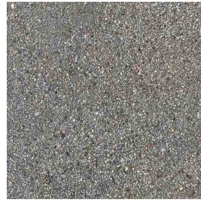
New Concrete Walks, Landings and Stepping Stones
