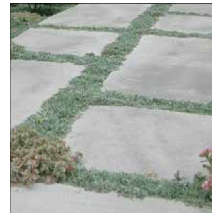
Concrete Pavers w/ Planting Strips
