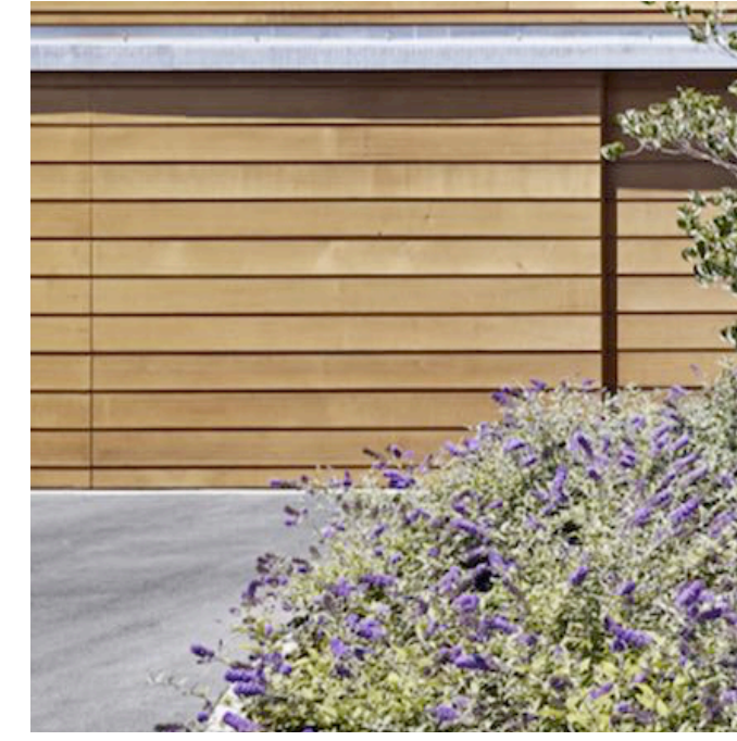
Exterior Wood Siding & Garage Door
