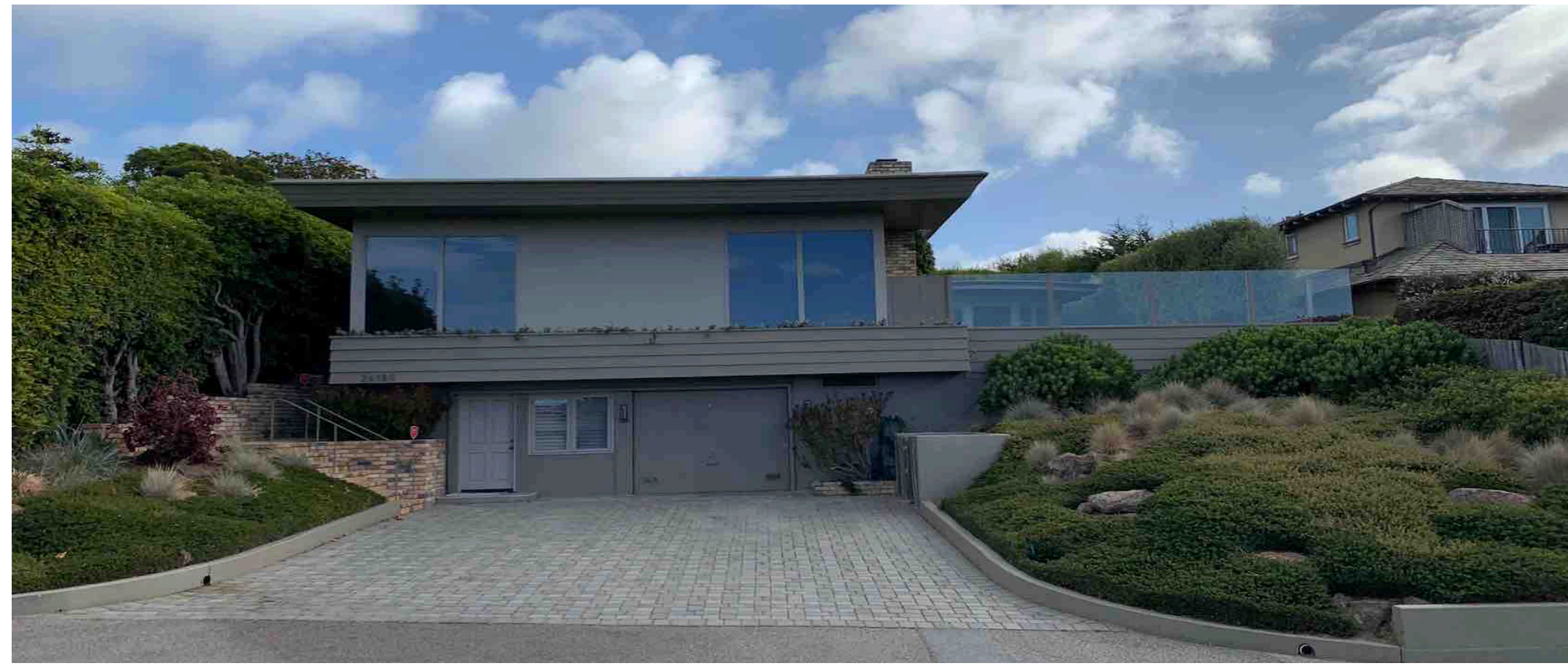
Existing View From Dolores Street
