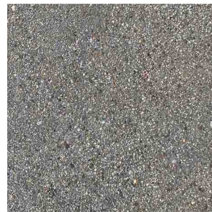
New Concrete Walks, Landings, and Stepping Stones
