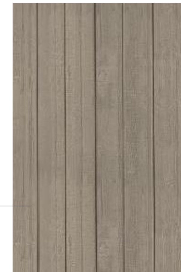
VERTICAL CEDAR SIDING (STAINED)
