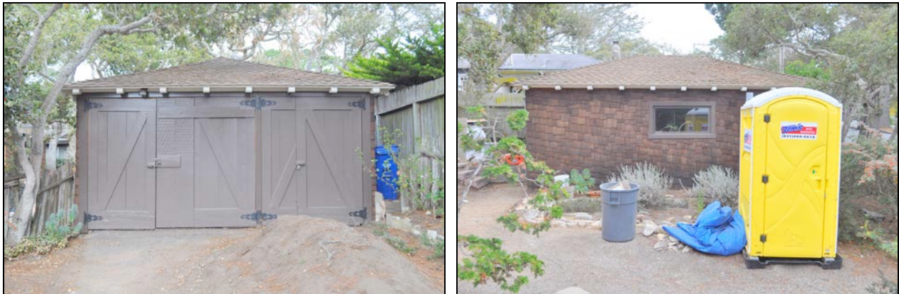
Figures 1 and 2. Left image shows the garage’s south elevation and the existing vertical-plank Redwood doors. Right image shows the garage’s west elevation, with fixed-sash window.
