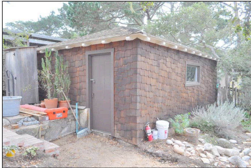
Figure 3. View of north and west elevations of garage.
