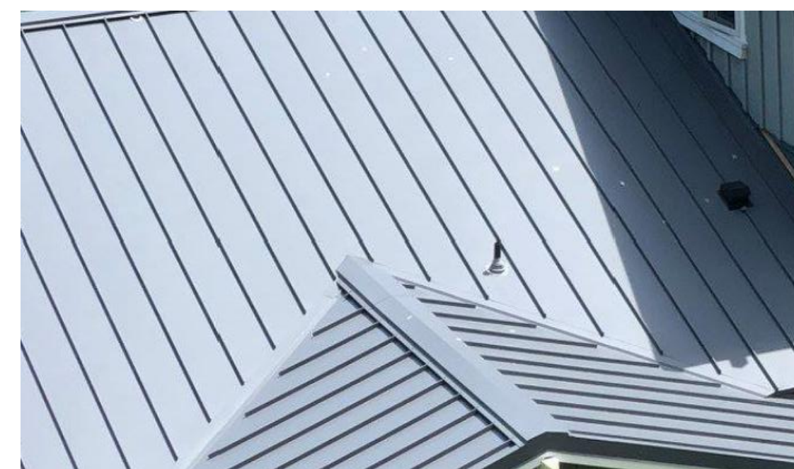
STANDING METAL SEAM ROOF
