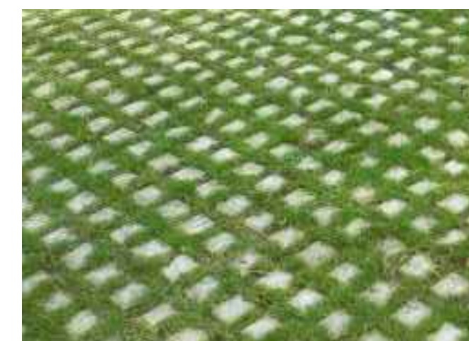
PLANTED PAVER DRIVEWAY
