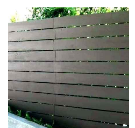
SIDE & REAR YARD FENCE - SPACED HORIZ. WOOD BOARDS TO MATCH WOOD SIDING ON HOUSE, FENCE WILL SLOPE TO MATCH SITE SLOPE
