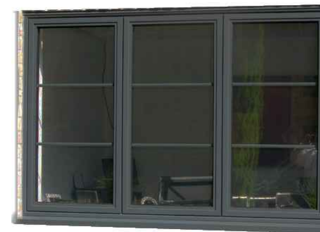
ALUM. CLAD WINDOWS & DOORS - DARK GRAY @ NEW WALLS
