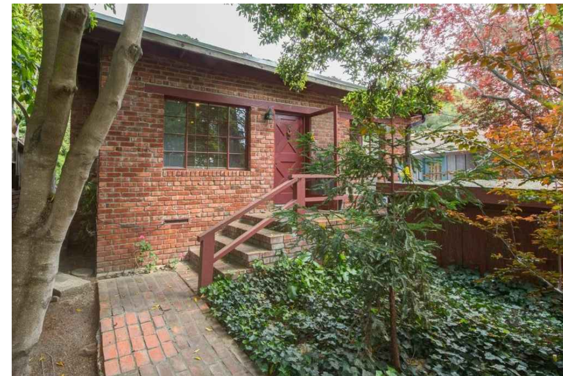
FRONT OF (E) HOUSE LOOKING EAST
