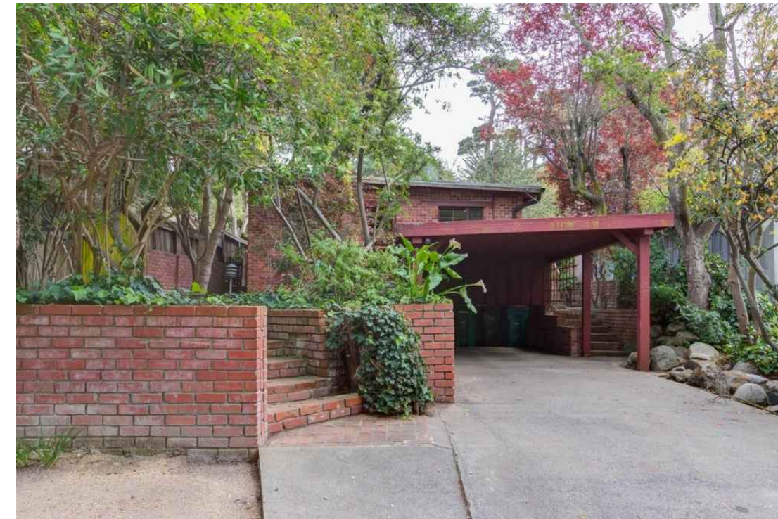
STREET VIEW OF (E) HOUSE LOOKING EAST
