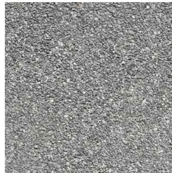
GRAY TAR & GRAVEL ROOF
