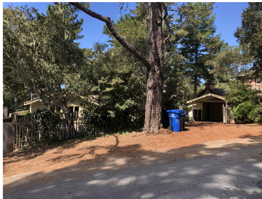
STREET VIEW OF (E) HOUSE & CARPORT
