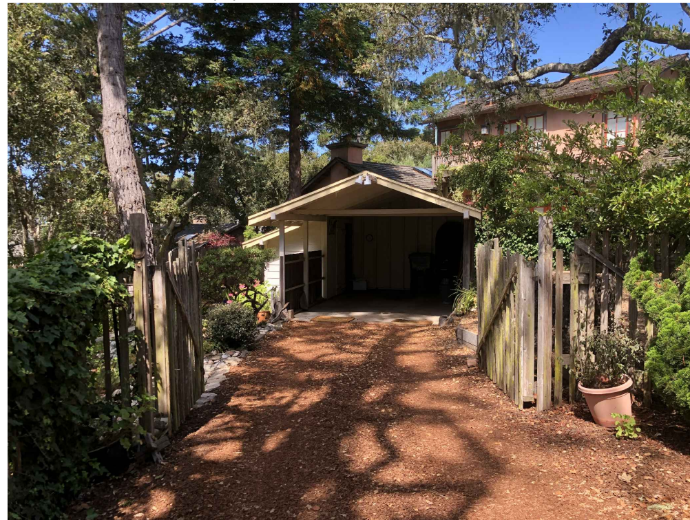
VIEW OF (E) CARPORT, LOOKING NORTHWEST
