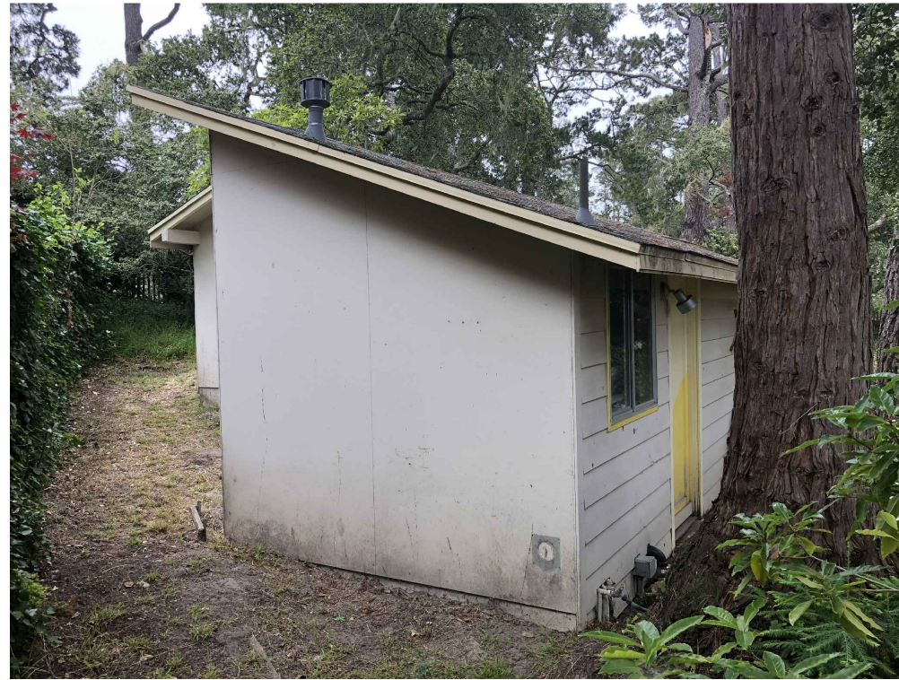
VIEW OF (E) CARPORT, LOOKING SOUTHEAST
