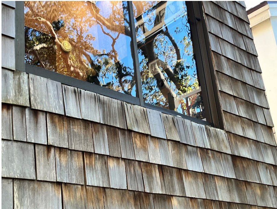
Figure 1: Views of damaged shingles
