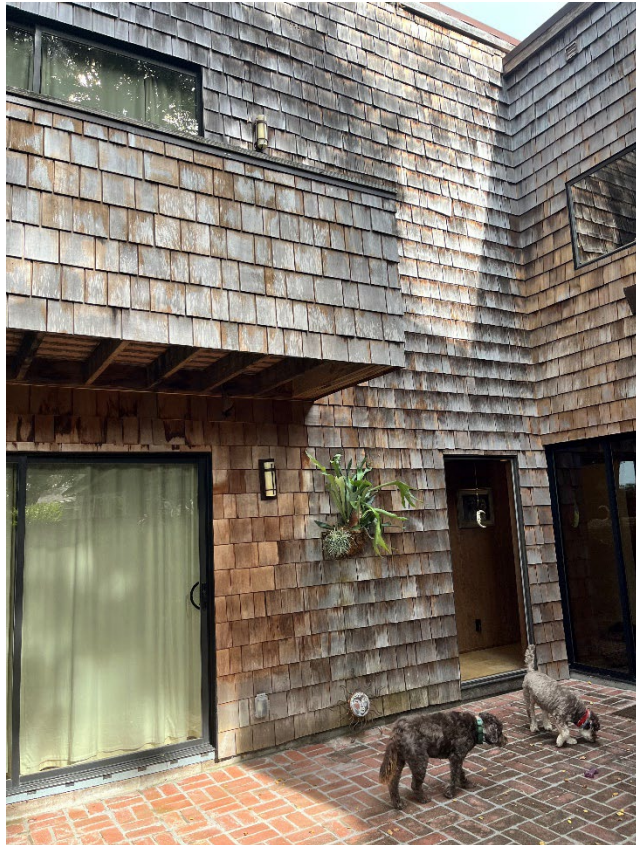
Figure 3: View of damaged shingles, west elevation.
