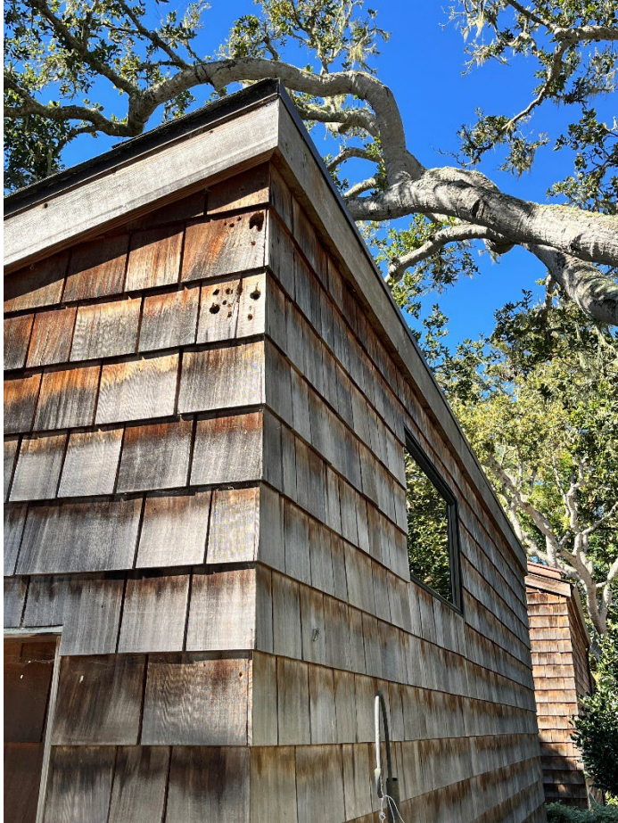
Figure 1: Views of damaged shingles
