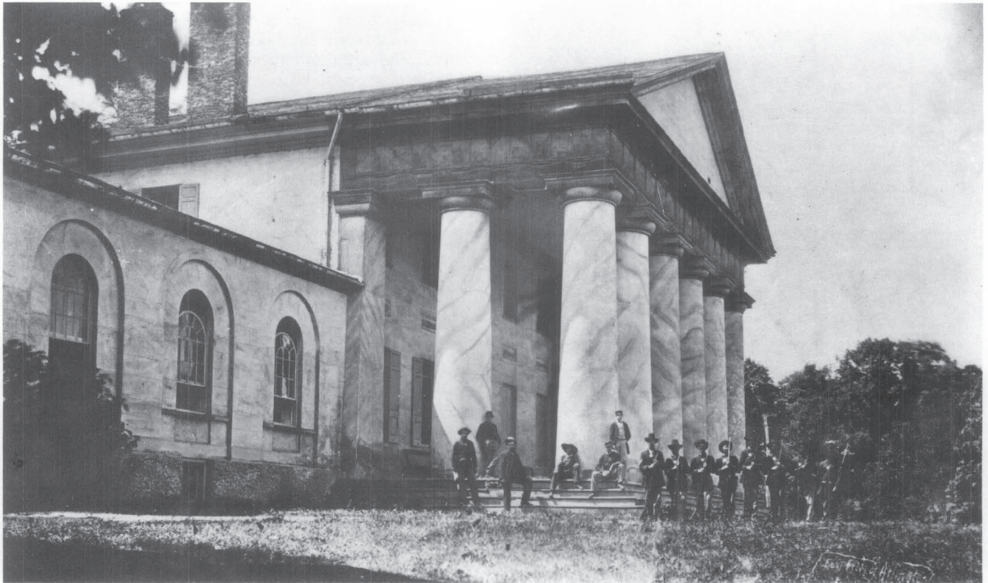
Fig. 6. Arlington House, Arlington, Virginia, was built between 1802–1818 of brick covered with stucco. It was designed by George Hadfield for George Washington Parke Custis, grandson of Martha Washington, and was later the home of Robert E. Lee. This photograph taken on June 28, 1864, by Captain Andrew J. Russell, a U.S. Signal Corps photographer, shows the stucco after it had been marbled during the 1850's. Yellow ochre and burnt umber pigments were combined to imitate Sienna marble, and the stucco, with the exception of the roughcast foundation, was scored to heighten the illusion of stone. Photo: National Archives, Arlington House Collection, National Park Service.
