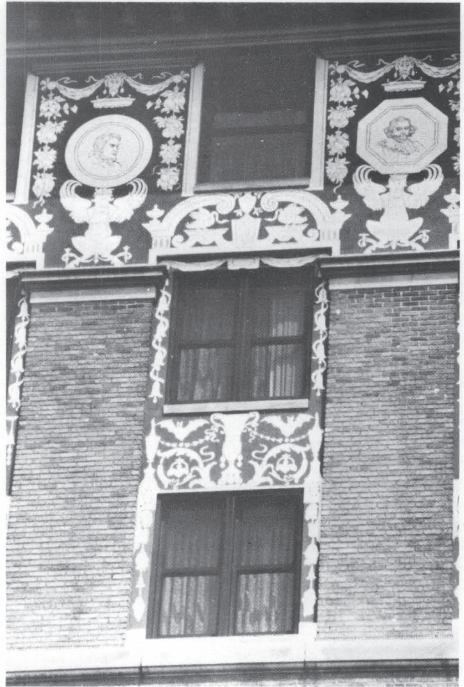
Fig. 11. The Hotel Washington, Washington, D.C. (1916–1917), is notable for its decorative sgraffito surfaces. Stucco panels under the cornice and around the windows feature classical designs created by artists who incised the patterns in the outer layer of red-colored stucco while still soft, thereby exposing a stucco undercoat of a contrasting color. Photo: Kaye Ellen Simonson.
