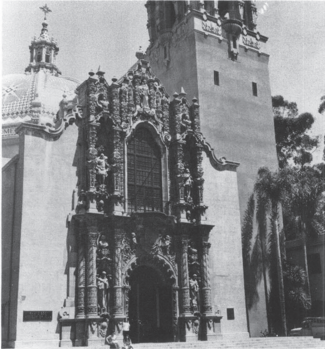
Fig. 4. The elaborate Spanish Colonial Revival style of this building designed by Bertram Goodhue for the 1915 Panama California Exposition held in San Diego's Balboa Park emphasizes the sculptural possibilities of stucco. Photo: C. W. Snell, National Historic Landmark Files.
