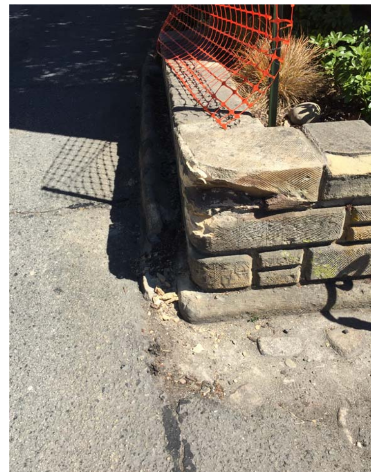
Typical damage caused by auto collisions into the base of the Monument
