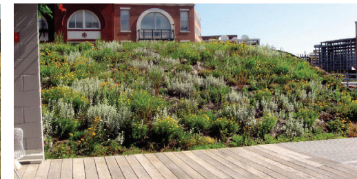
Extensive Garden Roof Assembly with Grasses, Groundcovers, and Shrubs
