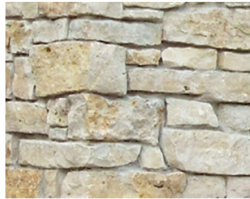
THIN VENEER STONE CLADDING
