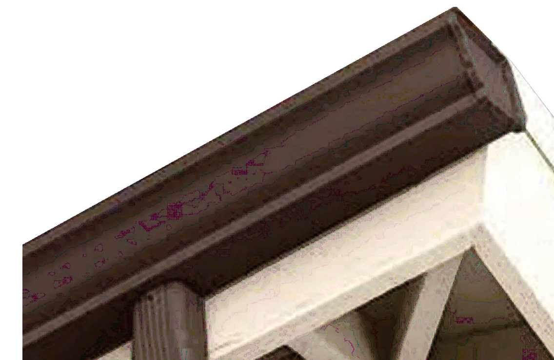
GALVANIZED BENT METAL GUTTER
