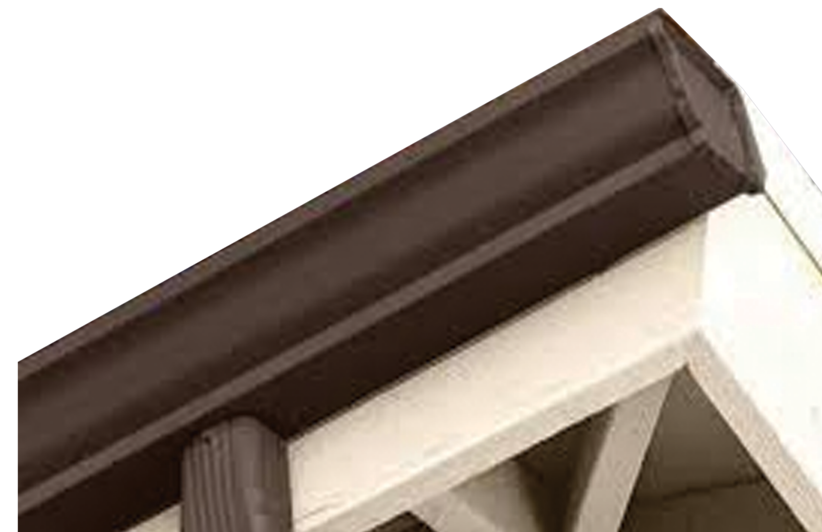
GALVANIZED BENT METAL GUTTER
