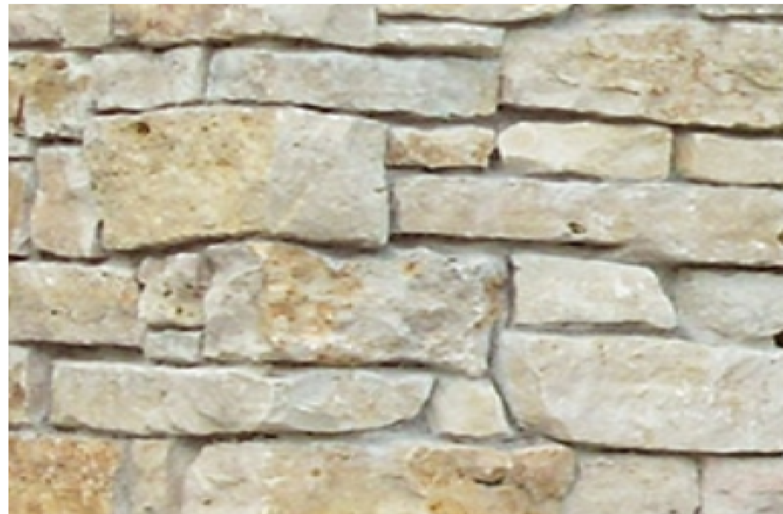
THIN VENEER STONE CLADDING
