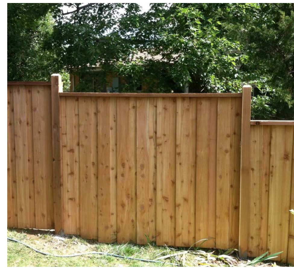
6' WOOD PRIVACY FENCE WITH GATE STAINED VERTICAL WOOD SLAT NORTH YARD ONLY, REPLACES EXISTING GATE
