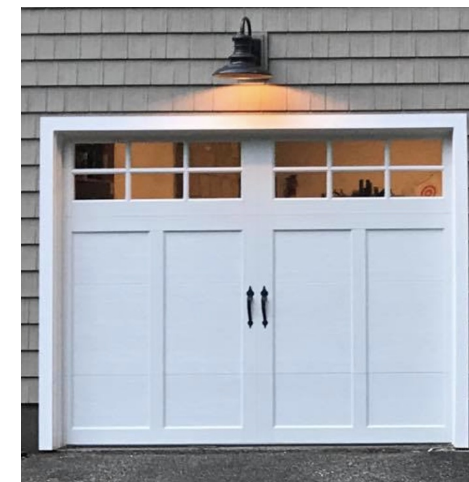
GARAGE DOOR STEEL - SIMULATED WOOD GRAIN TRUE DIVIDED LITES PAINTED SHERWIN WILLIAMS WHITE SNOW SW9541
