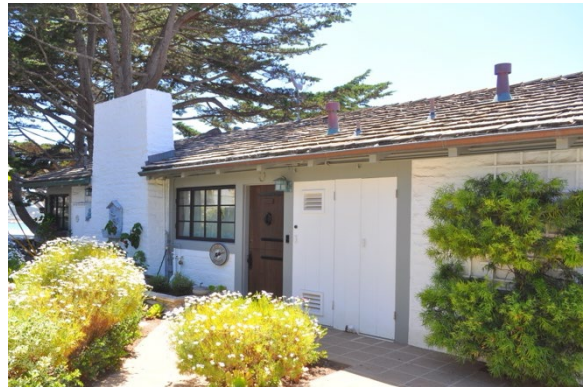
Post-Adobe House (1950), Scenic Rd. and 8 th Ave.
