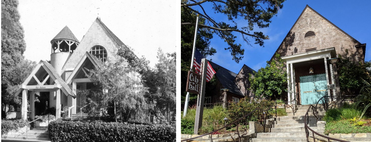
Left: Circa-1930 image of All Saints Episcopal Church (1913) after the M.J. Murphy additions ( Source: Kent L. Seavey Archives ). Right: 2024 image of City Hall ( Source: Past Consultants, LLC, 2024 ).
