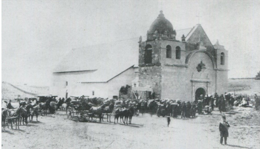
C.W.J. Johnson photograph of the August 28, 1884 rededication ceremony for the Carmel Mission, showing the replaced roof of improper pitch, compared to the original design (Source: Carmel: A History in Architecture ). 62
