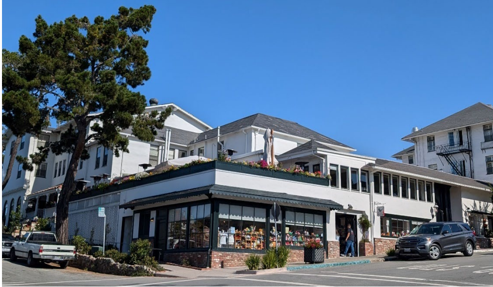
The Pine Inn (1889). (Source: PAST Consultants, LLC, 2024)
