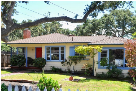
California Ranch house (1941), south side of 4th Avenue between Lobos St. and Randall Way
