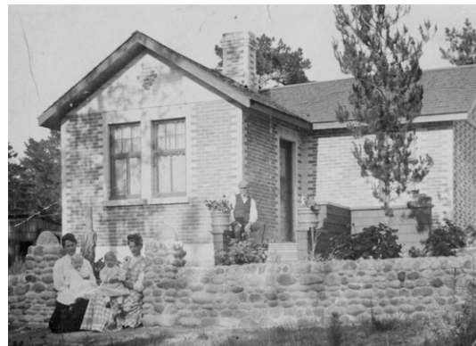
Benjamin Turner House (1898), Monte Verde St. 3 SE of 5 th Ave. 67
