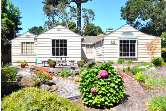
Unit House (1934), Torres 4 NW of 8 th
