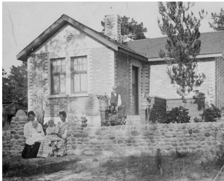
Circa-1900 image of the Benjamin Turner House, showing its vernacular-styled gable-on-wing massing, albeit with brick, rather than wood, wall cladding (Source: Henry Meade Williams Local History Department, Harrison Memorial Library ).
