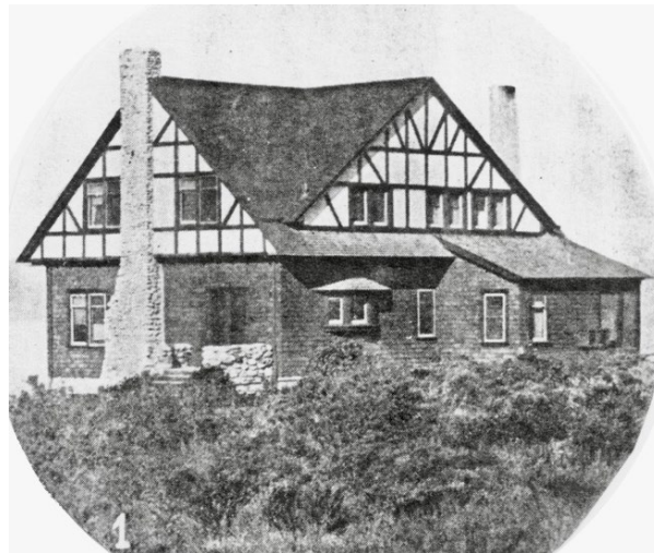
Early image of Grace McGowan Cook House (“Locksley Hall”)(1905) designed for the writer Grace McGowan Cooke and her sister Alice McGowan, extant on the north side of 13 th Ave between San Antonio Street and Carmelo (Source: Carmel: A History in Architecture ).
