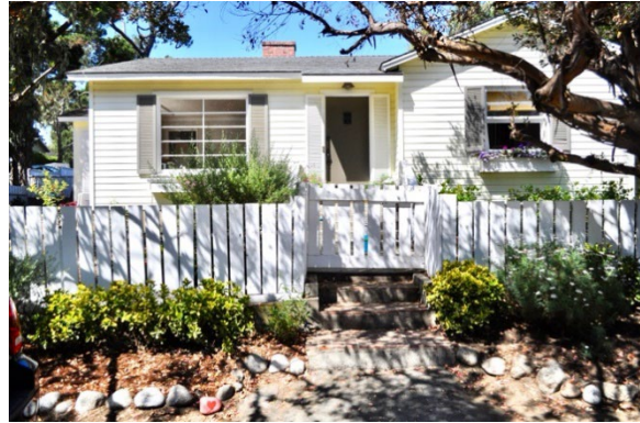
Adrian W. McEntire House (1939), NW corner of Mission and 11 th
