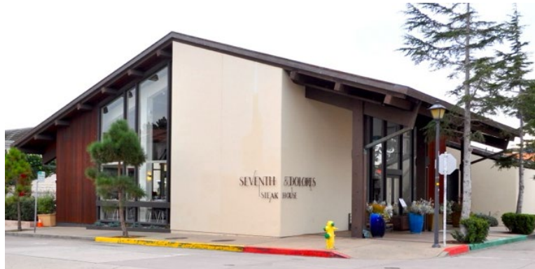
Northern California Savings and Loan (1972) by Burde Shaw Associates on the southeast corner of Dolores Street and 7 th Avenue (Source: PAST Consultants, LLC 2024).
