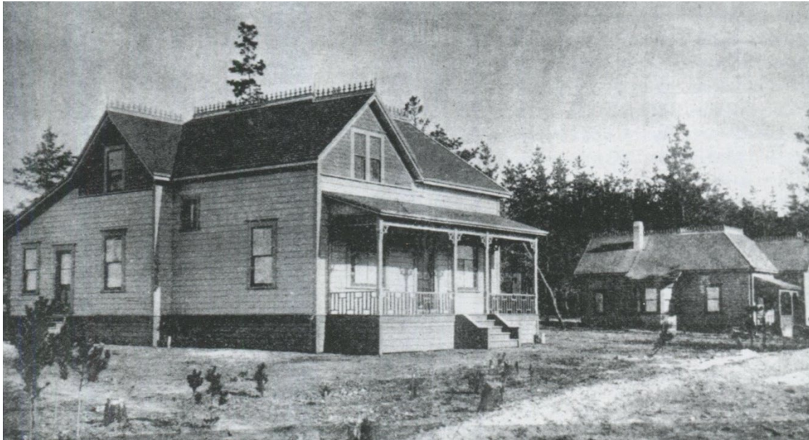
Historic image of the circa-1894 Abbie Jane Hunter house (right) and the Augusta Robertson house (left, demolished) constructed by Delos Goldsmith, likely from pattern book designs (Source: Carmel-By-the-Sea: Images of America ). 57
