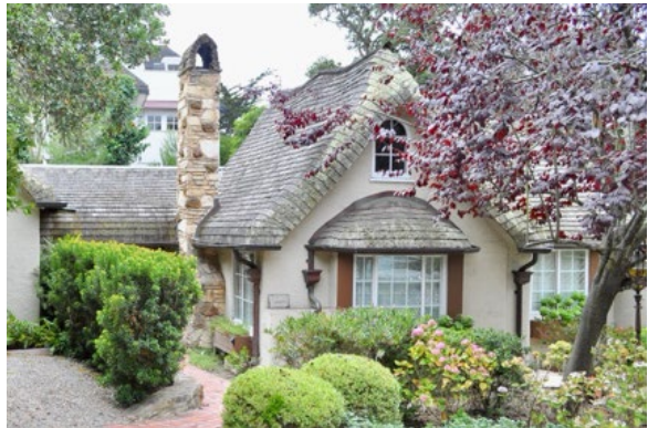
Grant Wallace Cottage (1927), southeast corner of Torres and 6 th
