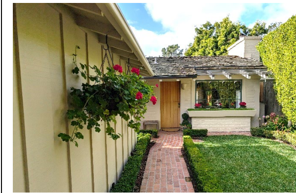
L.L. Spillers Guest Cottage (1951), Carpenter 4 SW of 3 rd Ave.
