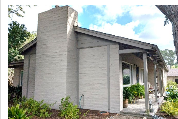
Post-Adobe House (1950), Vizcaino Ave. and Flanders Way
