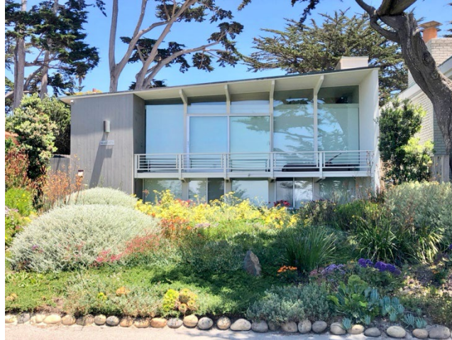
Clarence Mayhew's Helen Proctor House (1953) on Scenic Rd. 2 NE of 13 th (Source: PAST Consultants, LLC, 2024 ).
