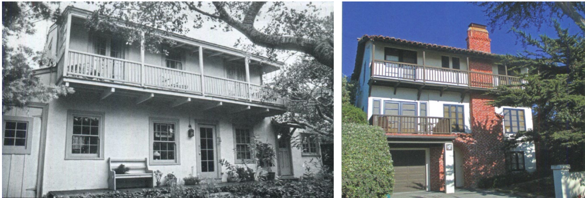
Left: The Kluegel House (1922) on Camino Real 4 NE of Ocean (Source: Kent L. Seavey Archives). Right: E.H. Cox House (1930) on Scenic 2 NW of 9 th Avenue (Source: Historic Homes and Inns of Carmel-by-the-Sea, 2016 ).
