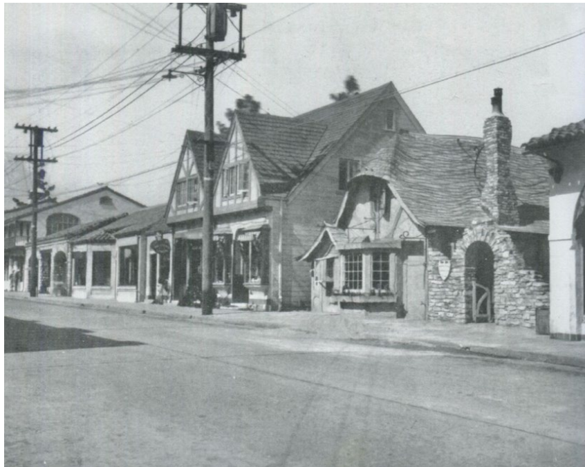
East side of Dolores Street, between Ocean and 7 th , circa-1931. From left to right: Isabel Leidig Building (1925); W.C. Farley Building (1927); Vining's Meat Market (Percy Parkes Building - 1926); De Yoe Building (1924); Tuck Box (1926); and a portion of the El Paseo Building (1928). Source: Pat Hathaway Collection, Monterey County Historical Society.
