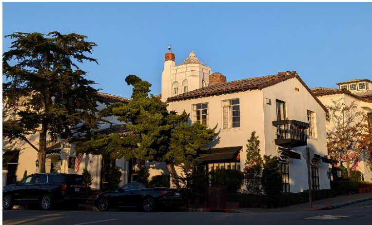
Left: Cypress Inn (1929) at the northeast corner of Lincoln St. and 7 th Ave, view of 7 th Street elevation prior to second-story addition by Gardner Dailey at the southwest corner of the building, shown in current image at right. (Source: PAST Consultants, LLC, 2024).
