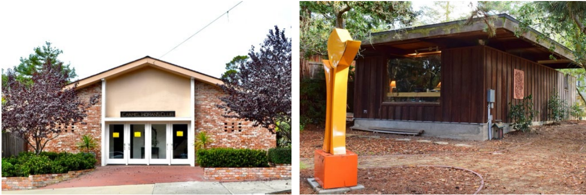
Left: Carmel Woman's Club (1948), southwest corner of San Carlos St. and 9 th Avenue (Source: PAST Consultants, LLC, 2024). Right: Paffard K. Clay's detached addition (1953) to the Carl Cherry Center (Source: Kent L. Seavey Archives).
