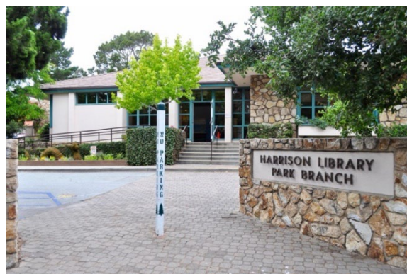
Harrison Library, Park Branch (1971), on the northeast corner of Mission Street and 6 th Avenue (Source: PAST Consultants, LLC 2024 ).
