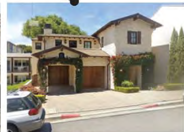
Brigantino Apartments - Rehabilitation of existing residential units.
