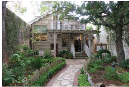
Der Ling Apartment - Conversion of commercial to residential use.
