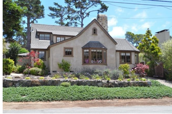
M.J. Murphy Office, west side of Monte Verde between 8 th and 9 th
