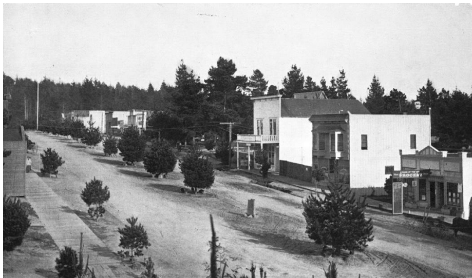
Circa-1910 image of the south side of Ocean Avenue, taken from the roof of the Pine Inn looking southeast. The Louis S. Slevin false front store (demolished) is at the center of the image, with the two-story Schweinger Building (extant, now the Carmel Bakery) to the right (Source: Harrison Memorial Library).
