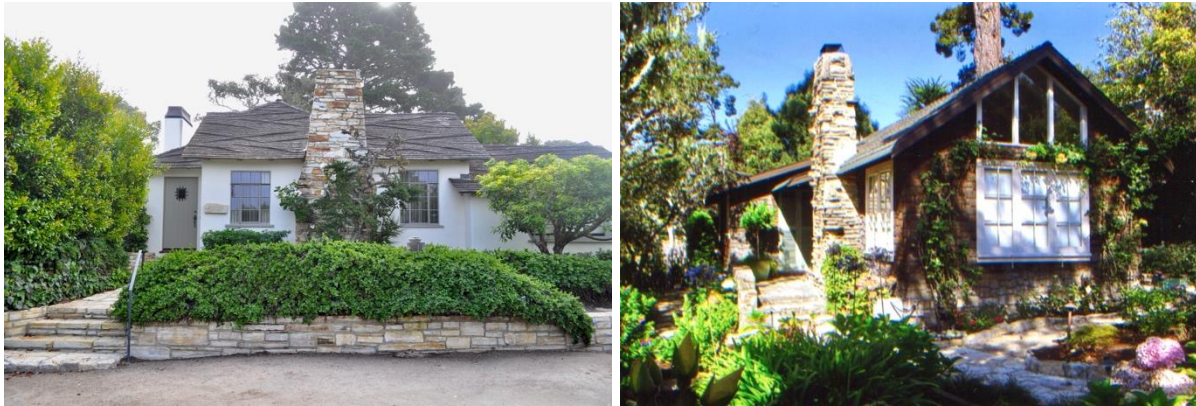
Left: Ernest Bixler's Alice Elder House on Camino Real Street 4 SE of 10 th Avenue. Right: Percy Parkes' Lollygag Cottage (Source: PAST Consultants, LLC, 2024).
