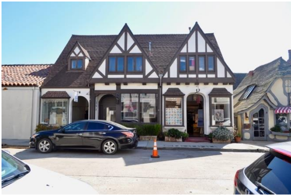
De Yoe Building, west side of Lincoln between 5 th and 6 th
