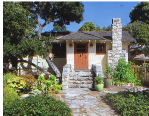
Carmel Cottage, east side of Mission between 11 th and 12 th
