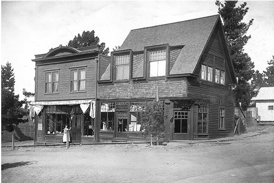
Historic image of the extant 1905 Shingle-style Philip Wilson real estate office at the northwest corner of Ocean Avenue and Dolores Street (Source: Carmel: A History in Architecture: Images of America , 46).
