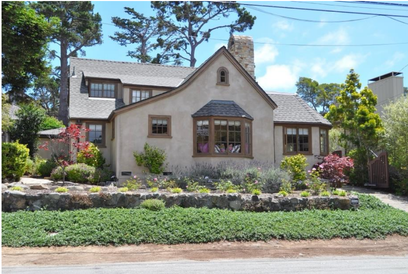
M.J. Murphy office on Monte Verde Street, 2 SE of 9 th Avenue (Source: PAST Consultants, LLC, 2024)
