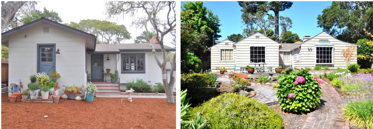
Left: Alta R. Jensen House by Edwin Lewis Snyder at Torres Street 5 NE of Eighth Avenue. Right: the Unit House by Hugh Comstock on west side of Torres Street, 9 South of Mountain View Avenue (Source: PAST Consultants, LLC, 2024).
