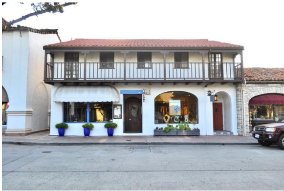
Isabel Leidig Building, east side of Dolores between Ocean and 7 th
