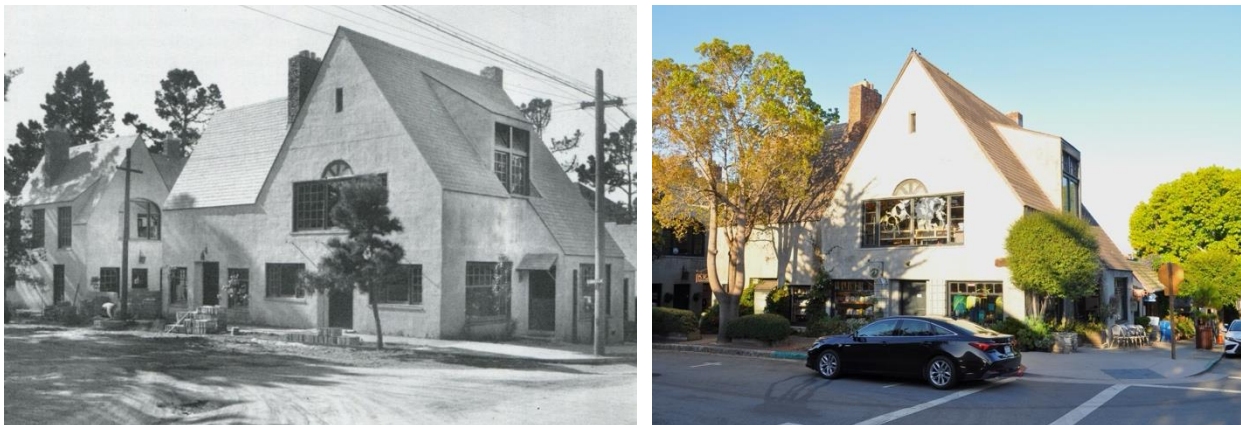
Left: Percy Parkes’s Thermotite-walled Seven Arts Building (1925), shortly after construction. Right: Current image of the Seven Arts Shop (Source: PAST Consultants, LLC, 2024).
