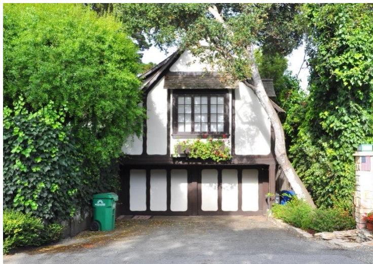
LaFrenz Garage/Studio on El Camino Real Street, 5 SW of 10 th Avenue (Source: PAST Consultants, LLC, 2024.)
