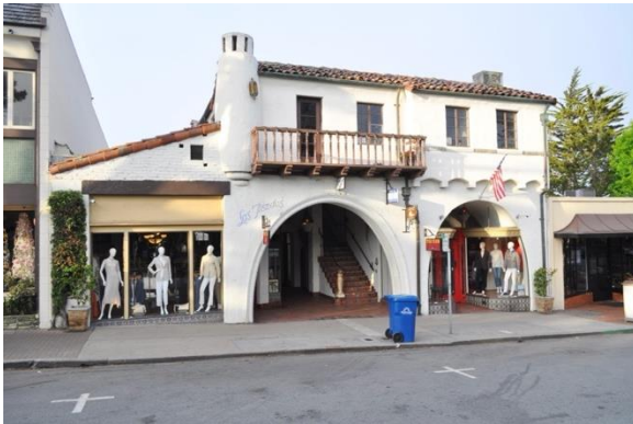
Las Tiendas Building, south side of Ocean between San Carlos and Dolores
