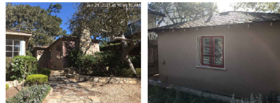
Front (South & West) Elevation (left) Rear (North) Elevation (right)
