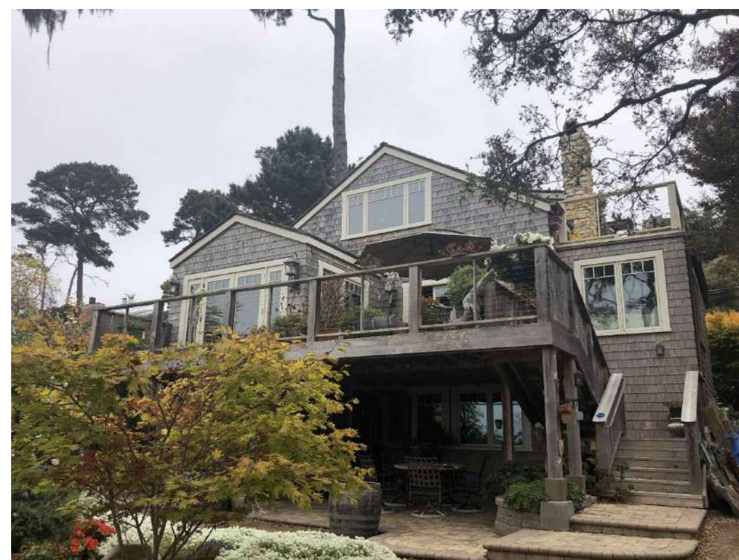
BACK OF HOUSE LOOKING NORTHEAST
