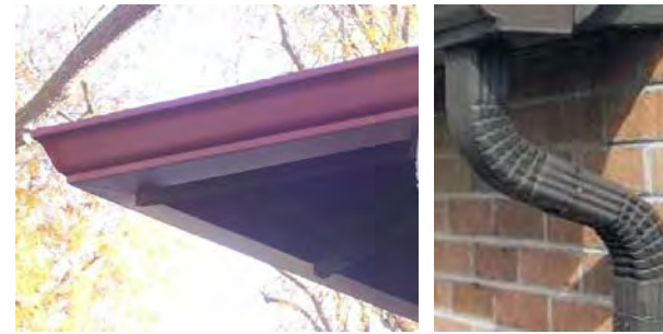
METAL GUTTER AND DOWNSPOUT (DARK BROWN, SOLID ALUMINUM)
