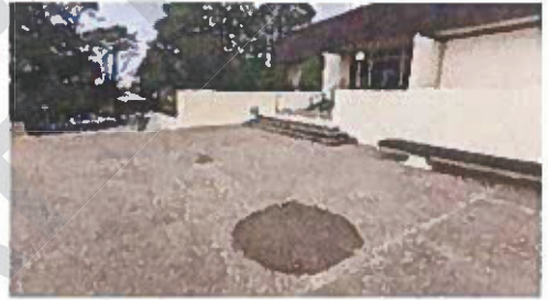
Figure 6 – Existing Garage Roof Paving
