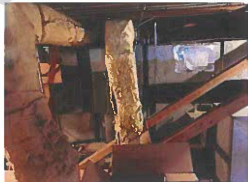
Figure 48 – Existing Duct Insulation
