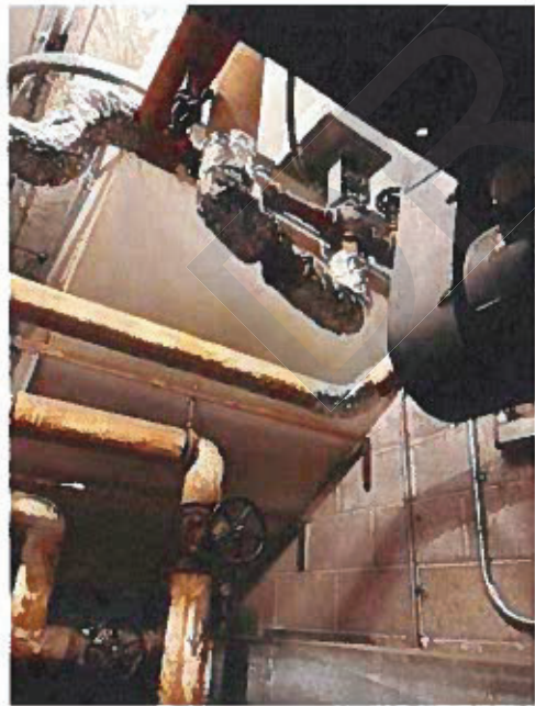
Figure 18 – Existing Hot Water Boiler (Mechanical Room)
