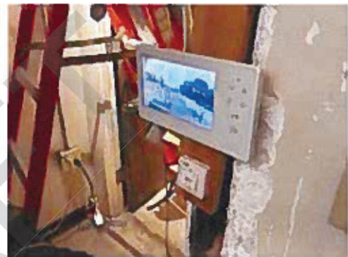
Figure 52 - Existing attic IDF with unsafe floor
