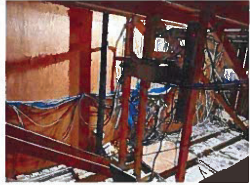
Figure 52 - Existing attic IDF with unsafe floor
