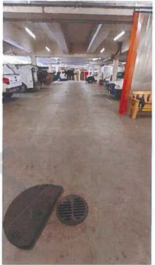
Figure 11 – Existing garage floor drains
