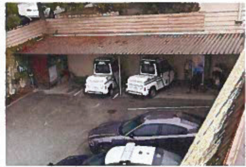
Figure 4 – View into Existing Non-Secure Patrol Covered Parking from Roof
