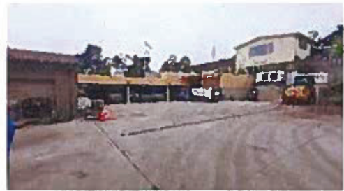
Figure 8 – Existing site paving
