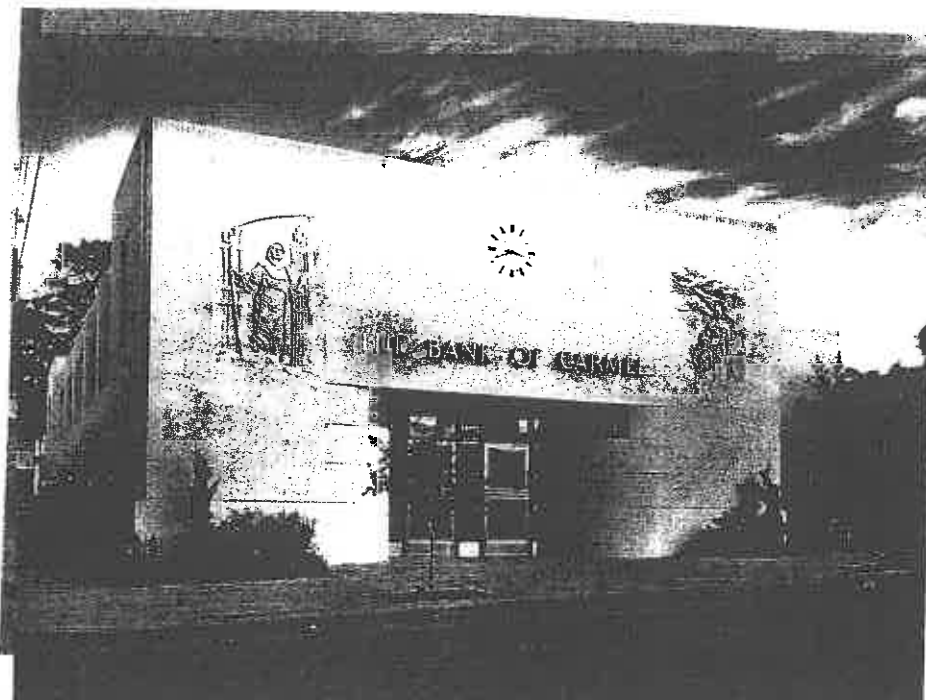
Looking North at South elevation, original entrance (1939)
