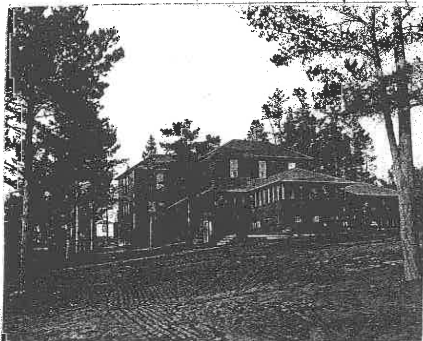
Looking N.E. at S/facing façade & W/side Elev. 1903, #73-14-4, Pat Hathaway, Historical California Views, Monterey
