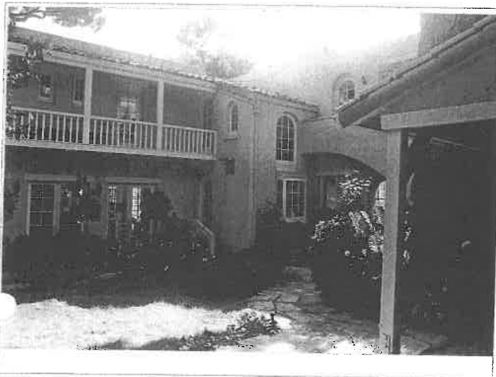
Description of Photo: (View, date, accession#) Looking SW at the interior courtyard. 9/1/01, #9183-26A
