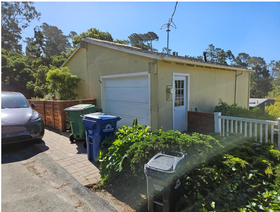
View of garage.
