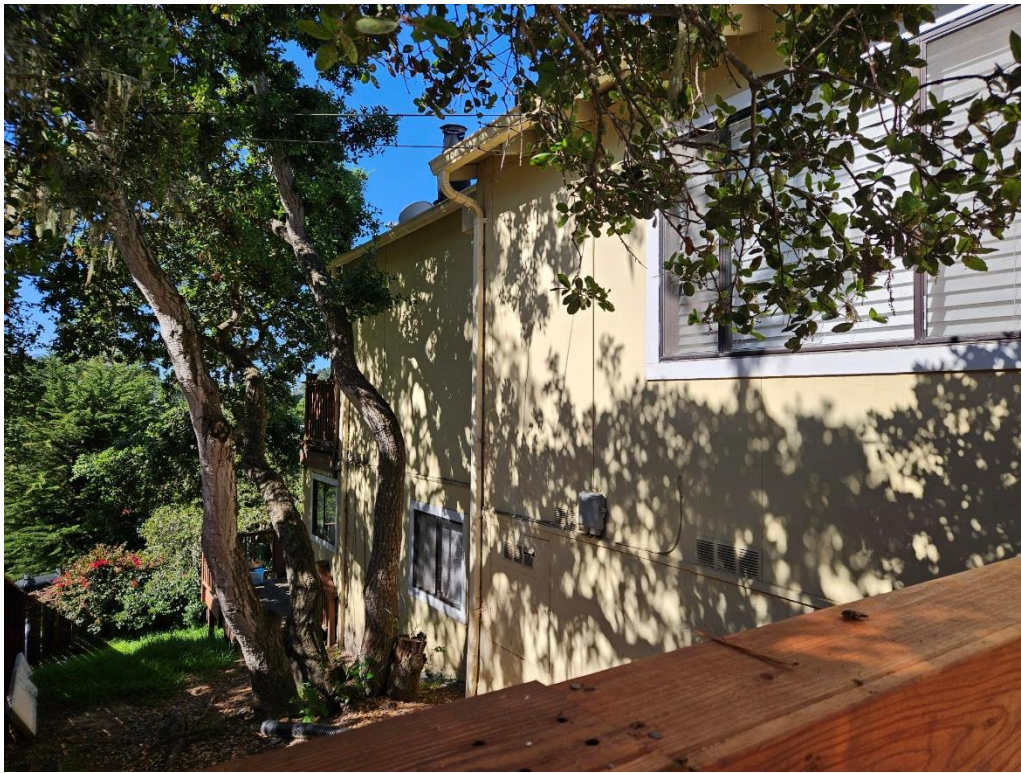
View of east elevation.
