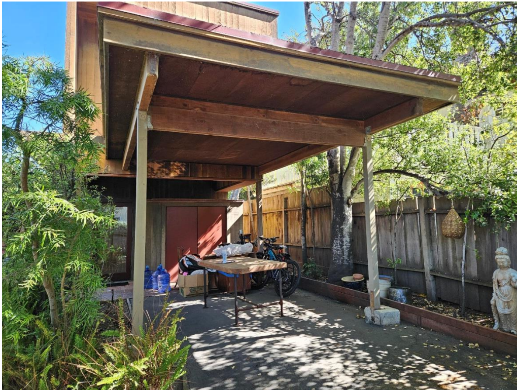
View of carport.
