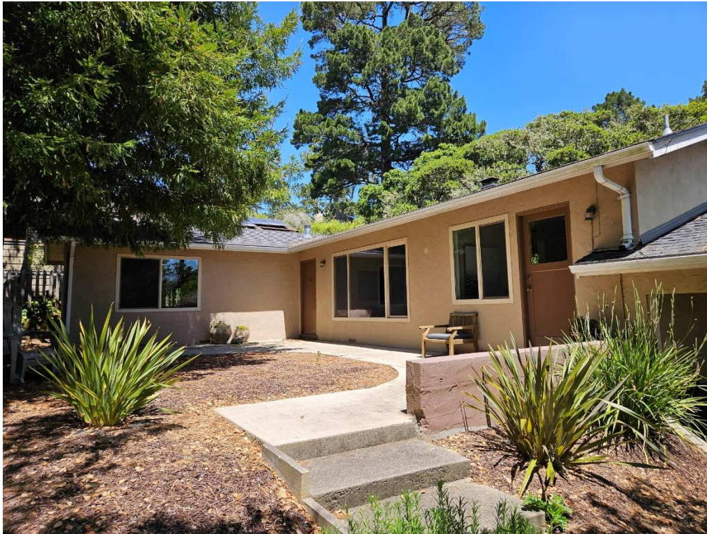
View of the house.
