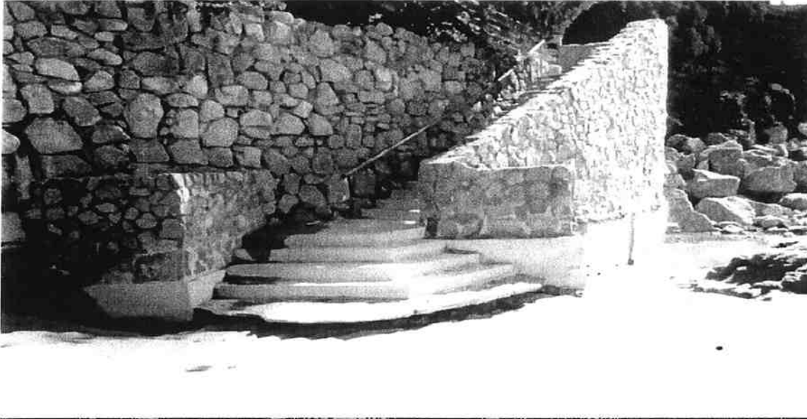
Photo 5 – The Tenth Avenue (South) Stairway
