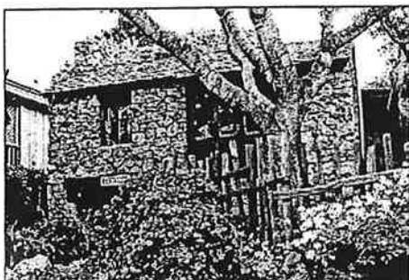
The construction method most often used was wood frame, although there were many homes constructed of rough cut stone.
