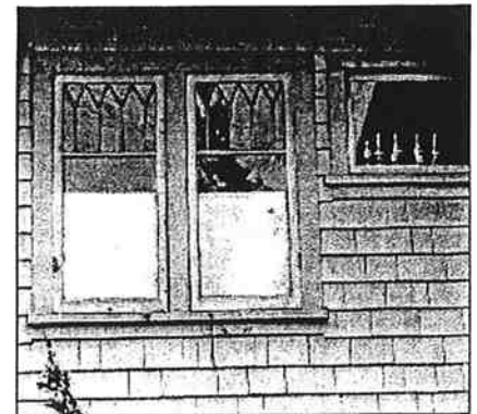
Vertically proportioned, double-hung windows appear on many buildings.
