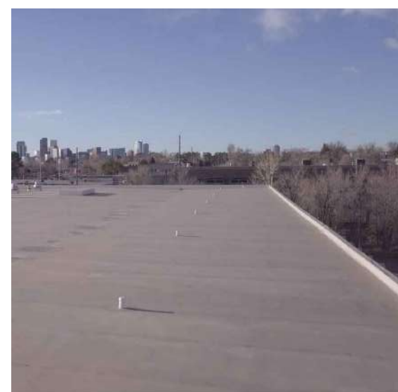
PVC ROOF MEMBRANE W/ GRAY GRAVEL SURFACING
