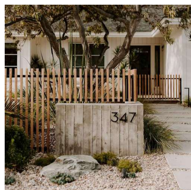
VERTICAL WOOD PICKET FENCE & GATE IN NATURAL FINISH, BOARD FORMED CONCRETE W/ TAN/BROWN PIGMENT
