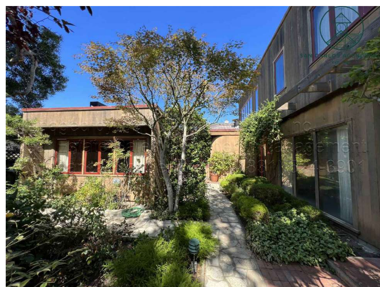
FRONT OF (E) HOUSE
