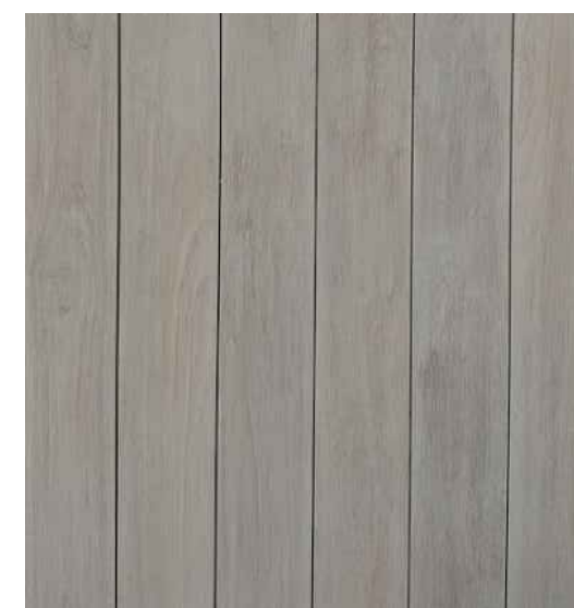
SAND & RE-STAIN (E) VERTICAL WOOD SIDING
