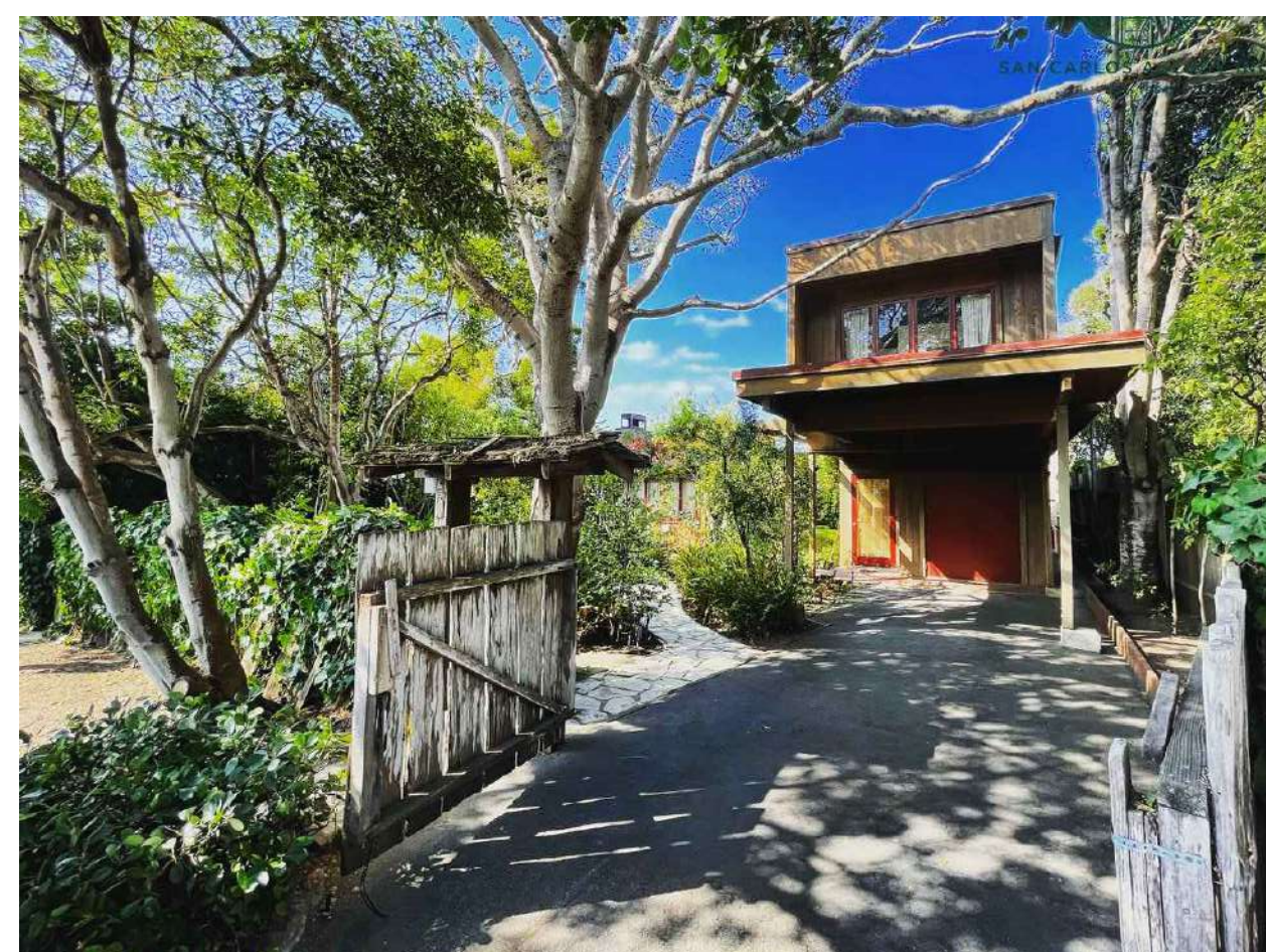
FRONT OF (E) HOUSE & CARPORT
