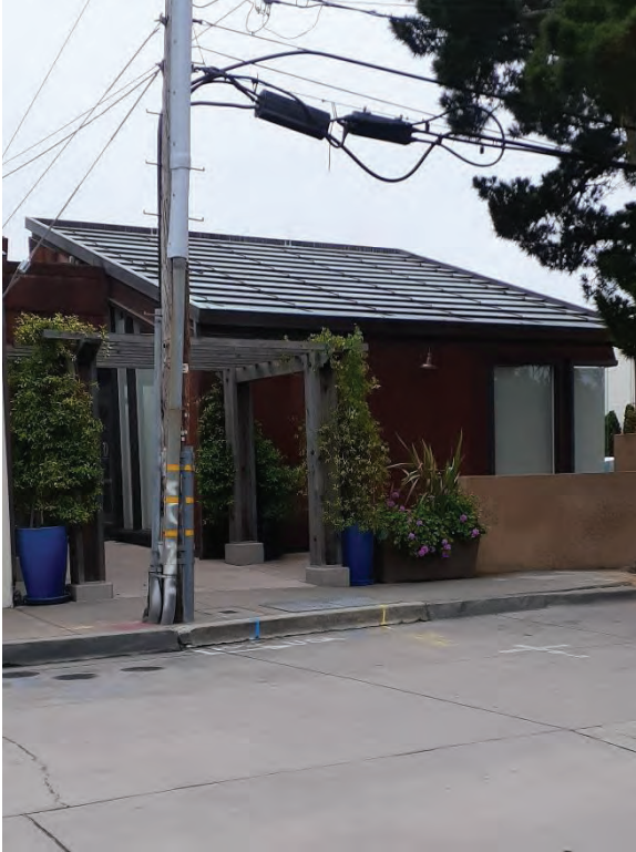
Front Elevation Facing Dolores Street, 2020
