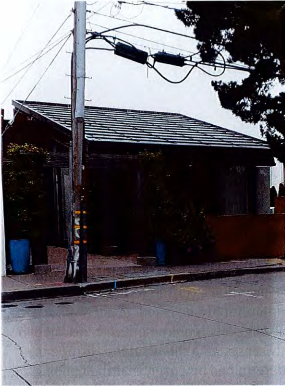
Front Elevation Facing Dolores Street, 2020
