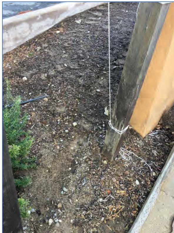
Figure 8: Soils exposed on the northwest corner of the project parcel.
