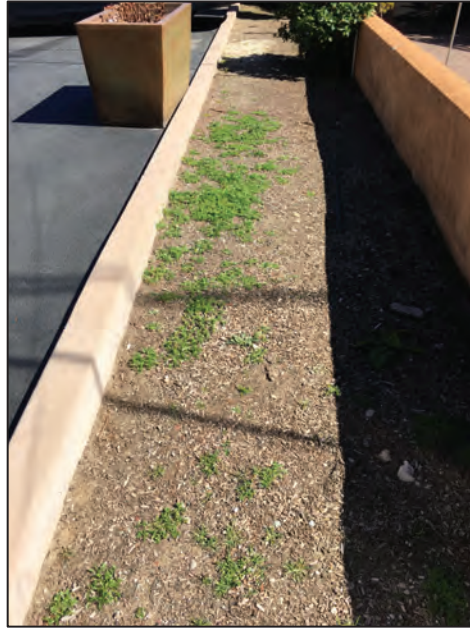
Figure 9: Soils exposed on the south side of the project parcel APN 010-145-024.
