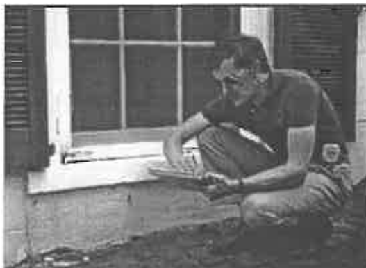
Window condition assessment preceding repair work.
