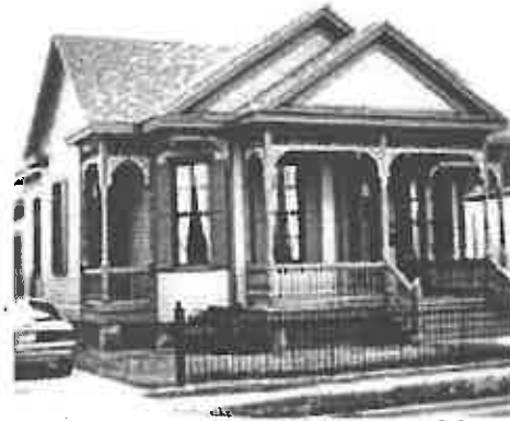
Porches repaired and painted as part of the rehabilitation work.
