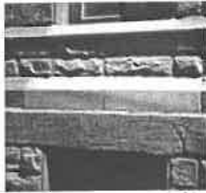
Replacement stones tooled to match original.
