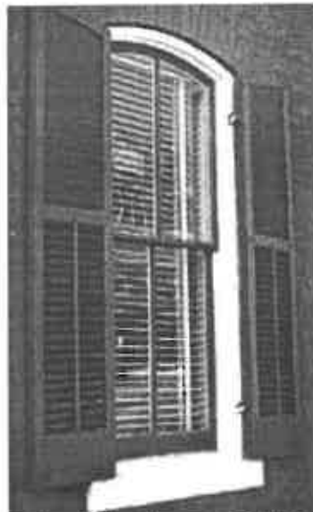
Well-maintained louvered shutters allow for ventilation and privacy.
