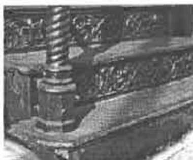
Cast-iron steps with distinctive cutout work.
