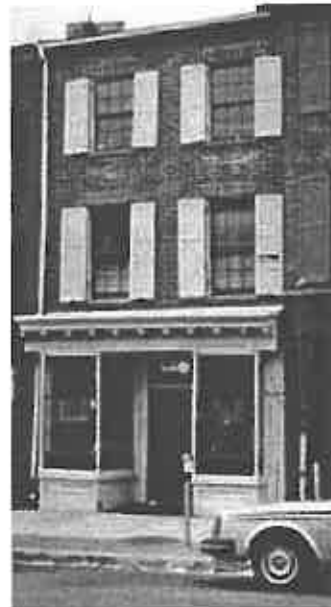
Distinctive 19th century brick and wood storefront in good repair.
