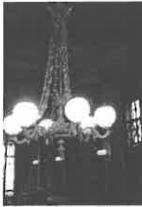
Ornate gas lighting fixture that has been electrified.
