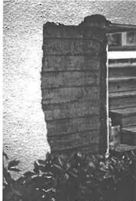
Preparation for stucco repair.
