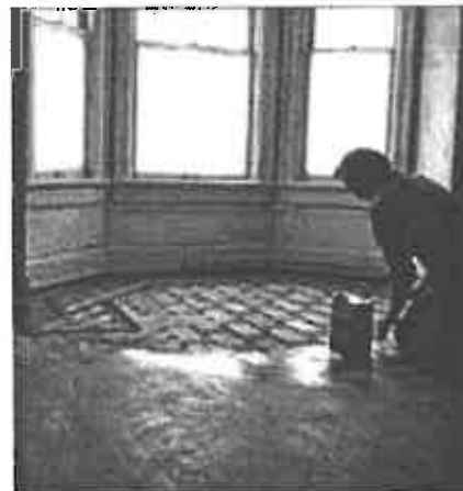
Applying a protective finish to historic flooring.
