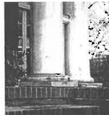
Replacing rotted wood column base with new wood.
