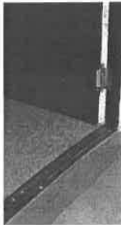
Historic threshold made accessible with 1/2" wood bevel.
