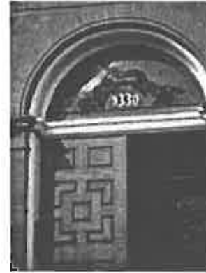
Stained glass arched transom characterizes entrance to 1880s rowhouse.
