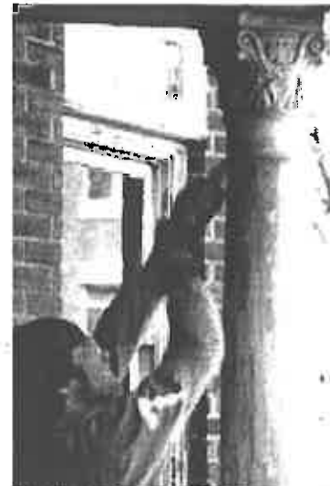
Hand scraping wood column prior to repainting.
