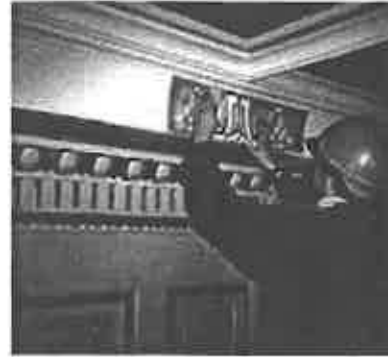
Painted interior finishes repaired during rehabilitation.
