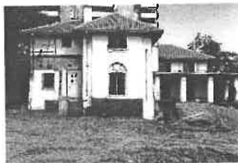
Important site features destroyed during rehabilitation.
