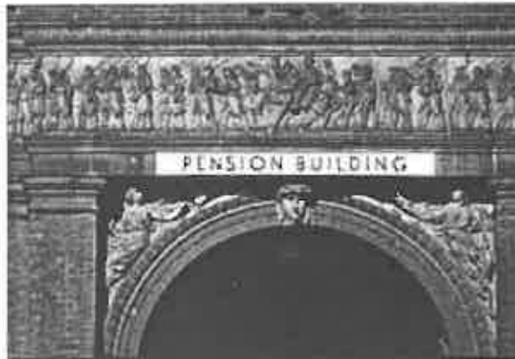
1880s brick building with terracotta trim.
