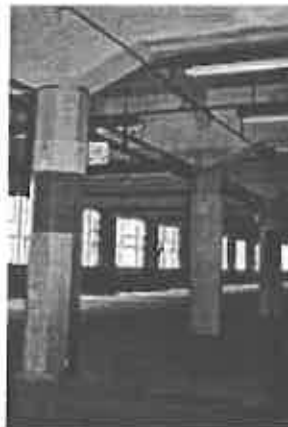
Reinforced concrete structural system in early 20th century industrial building.
