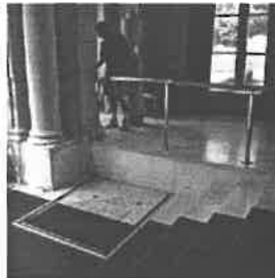
Compatible lift for historic foyer using "like" materials.
