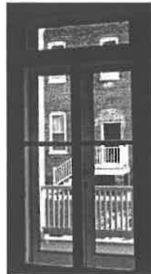
Storm doors added on inside of historic doors.
