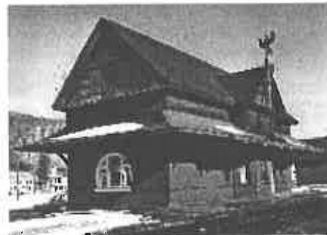
Gable and pent roof in excellent condition.
