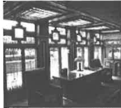
Restoration of lost features and finishes based on documentation.
