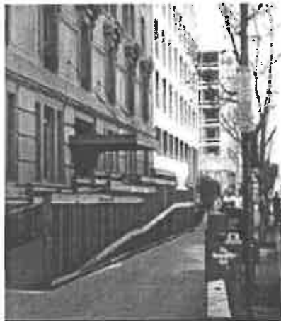
Large wood ramp incompatible with building's historic character.
