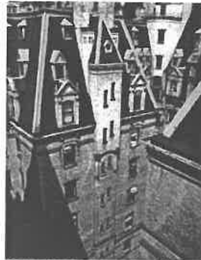
Slate and copper mansard roofs in an urban canyon.
