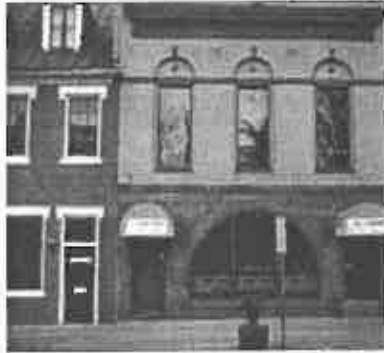
Incompatible replacement storefront and inappropriate window alteration.
