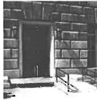
Entrance made accessible by adding inconspicuous ramp.
