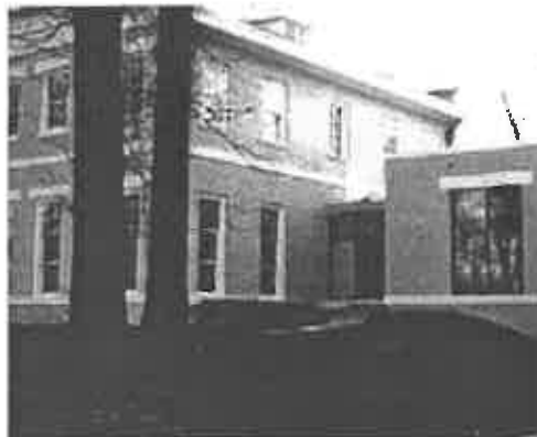
Compatible new addition on rear elevation of historic building.
