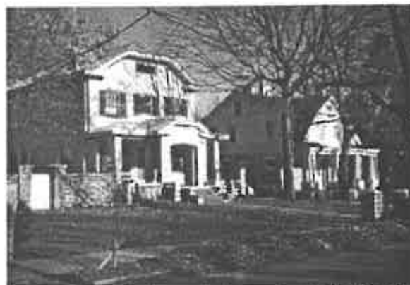
Deteriorated porch steps and stone garden wall replaced in kind to help unify a streetscape.
