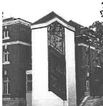
Large incompatible stairtower on highly visible elevation. Photo: Martha L. Werenfels, AIA.
