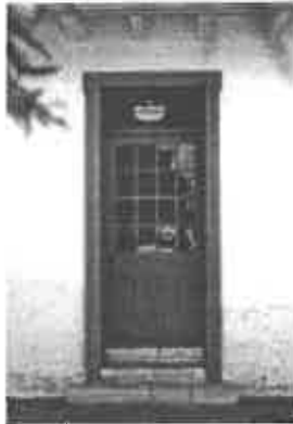
Operable over-the-door transom providing cross ventilation.
