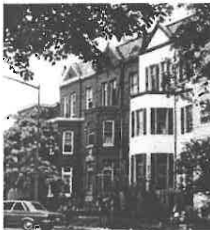
Urban setting marred by inappropriately altered house on right, now clad in vinyl siding.
