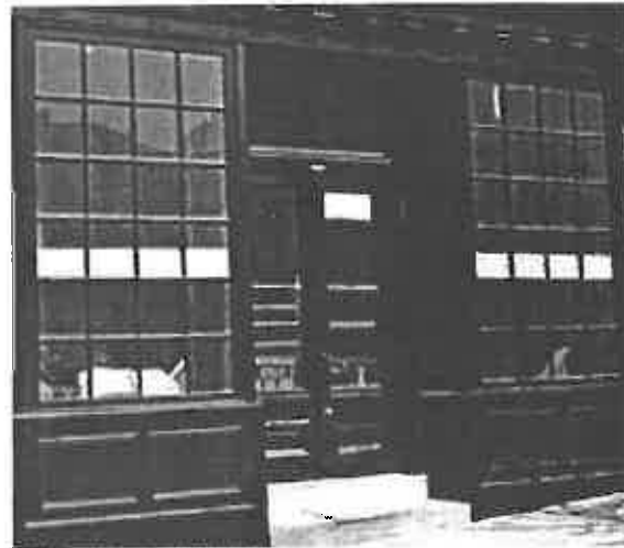
Well-maintained historic metal storefront.
