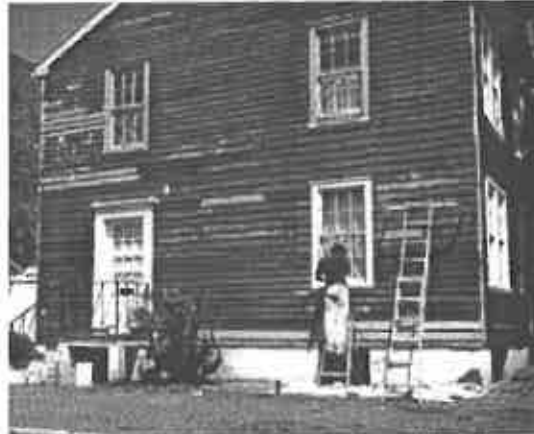
Limited replacement in-kind of deteriorated wood clapboards.
