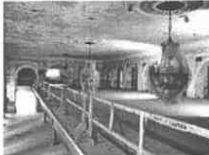
Spatial character of hotel lobby destroyed by inserting another floor level.
