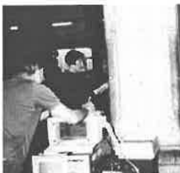
Using ultrasonic pulse velocity to determine thickness and soundness of solid granite column. Photo: Andrea Lazarski.
