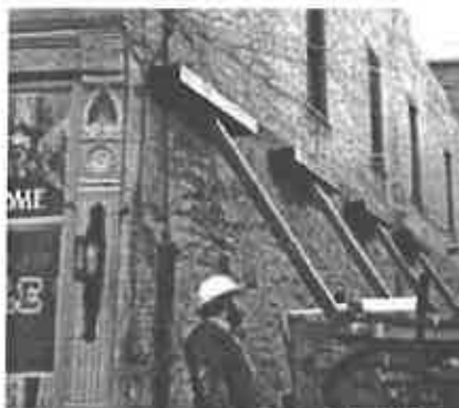
Structural stabilization of masonry walls before rehabilitation.
