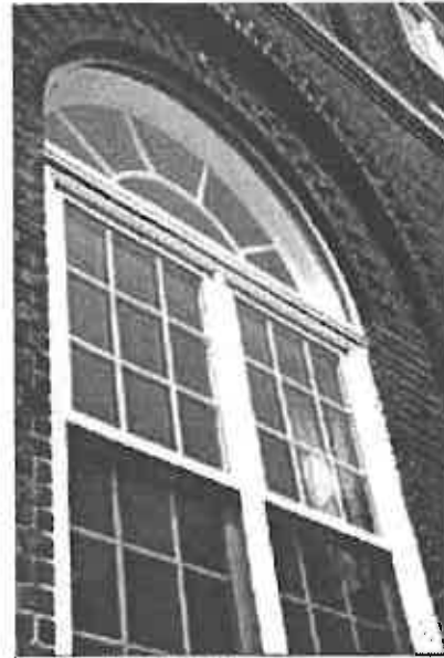
Newly painted double-hung wood windows.
