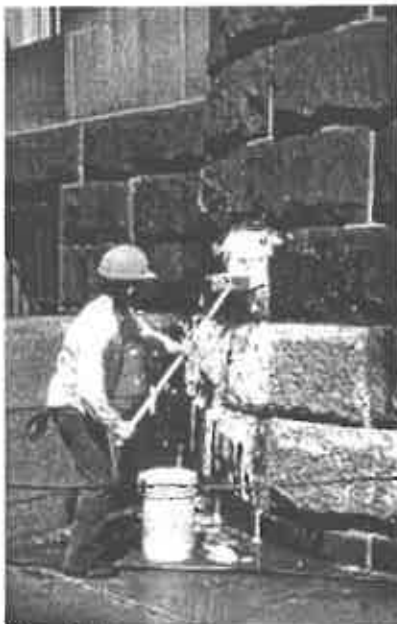
Chemical cleaning to remove dirt from granite.
