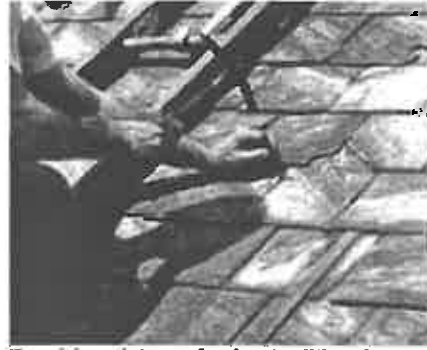
Repairing slate roof using traditional methods.
