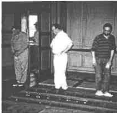
Evaluating floor joists prior to structural strengthening.
