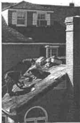
Insulating attic and installing replacement composition roof on 1920s house.
