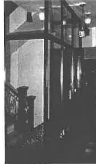
Enclosure that preserves decorative staircase and also meets safety code.
