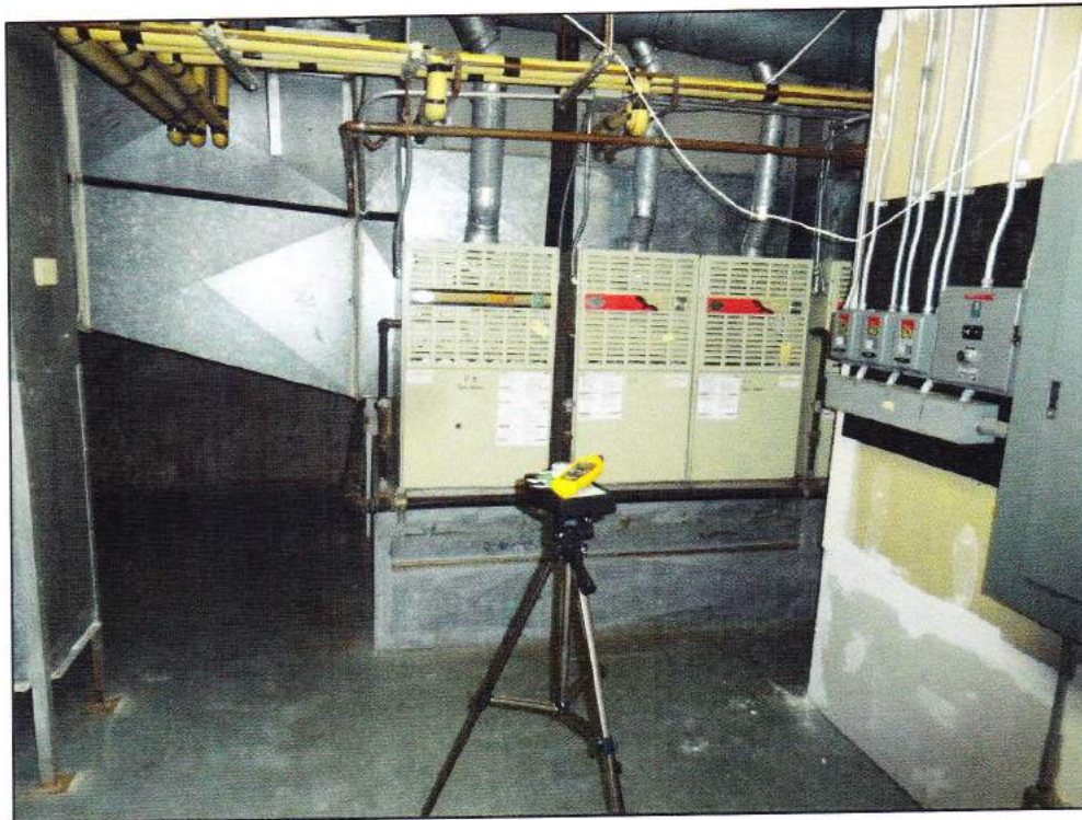
Sampling in mechanical room
