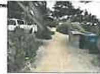
TRASH CONTAINERS: CONTAINERS HAVE CHANGED ORIGINAL SCREENED ENCLOSURE NOT PROVIDING THE INTENDED DESIGN SOLUTION
