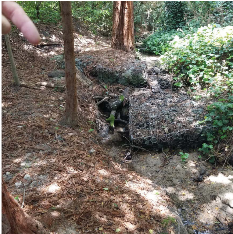
Photo 6: Looking Upstream at a failing gabion weir with a spillway that is undersized for even moderate storm events.
