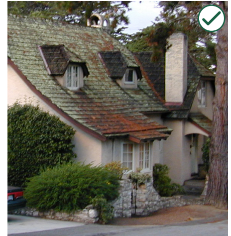
Appropriately sized dormers can be used to reduce scale and achieve a well-integrated design.
