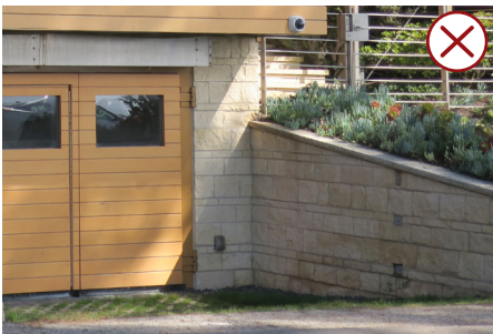
Large exposed retaining wall
