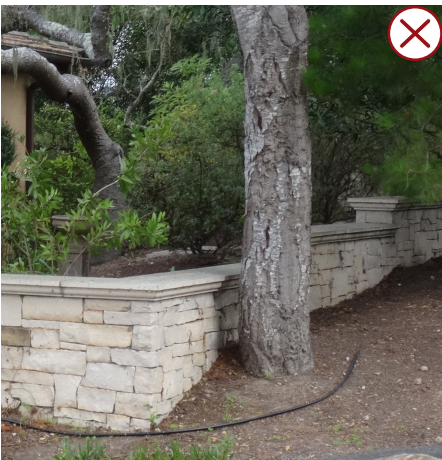
Avoid excavations or foundations that would cut into the root zone or drip-line around any significant tree.
