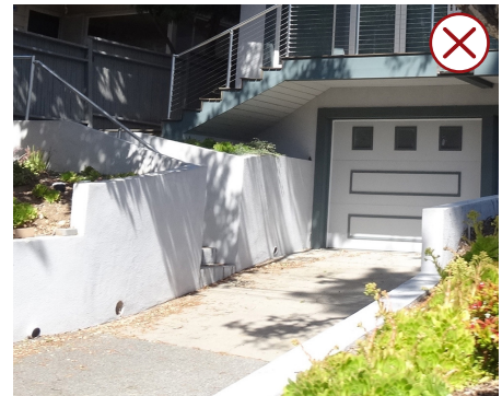
Large exposed retaining wall
