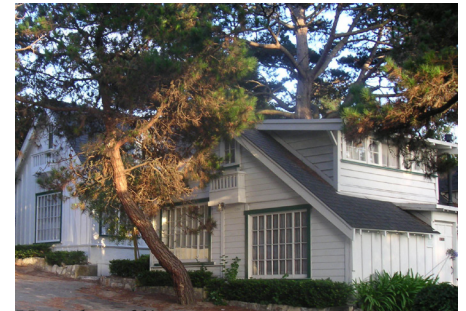
Varied roof lines
