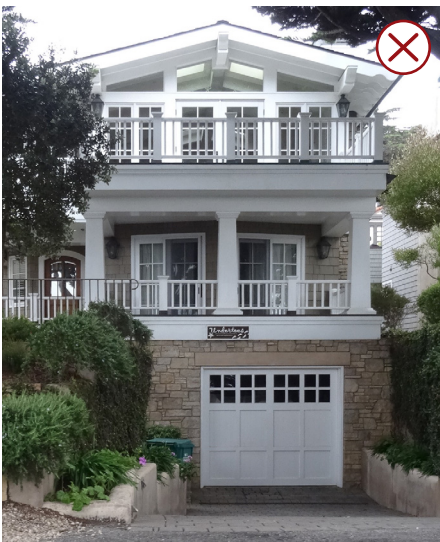
A building shall appear to be no more than two stories in height, as viewed from the public right-of-way.
