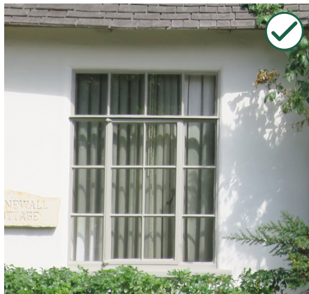
Multi-pane metal casement window
