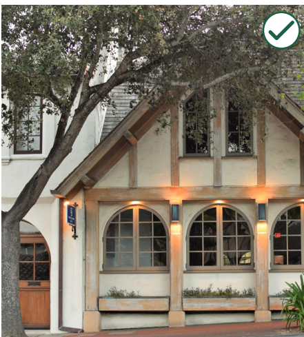
Traditional materials include wood, stone and stucco, all with matte finishes and in muted earth tones.
