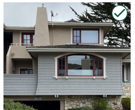
Use variations in surface treatments to convey traditional building scale in a facade.
