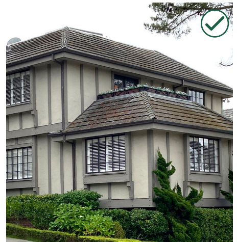
Stucco that is stained or painted and is either smooth or lightly textured is appropriate.
