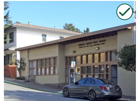
Avoid abrupt changes in grade on the site and between adjoining properties.
