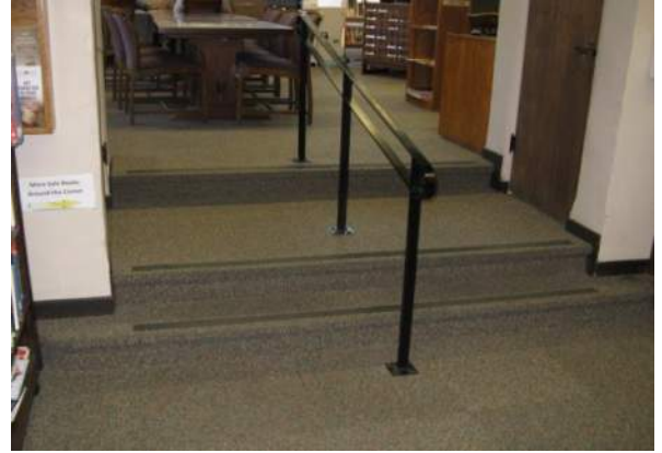
L. South Stair to Reference Department from Lobby
