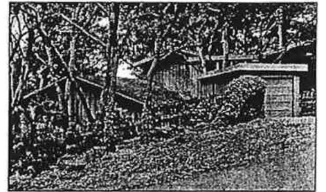
The community has experienced a series of design trends during its development. Underlying all these variations was a conscious intent of creating a village in a forest setting.
