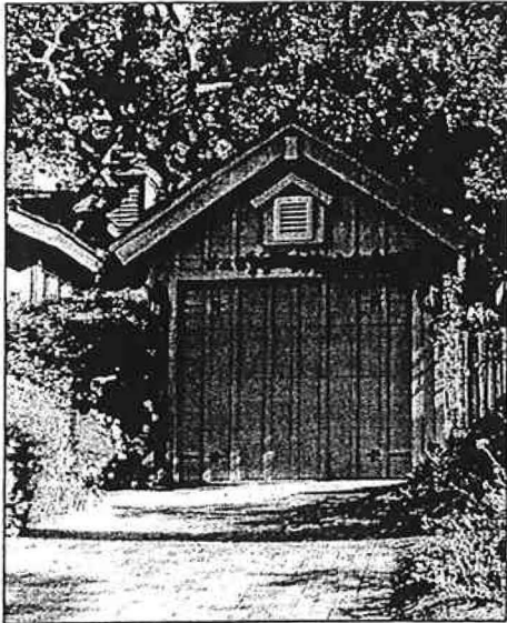
Preferred: This overhead door matches the board and batten siding of the garage itself.
