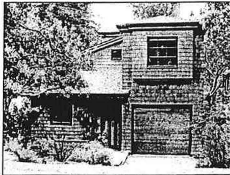
Preferred: This garage door blends with the house siding.
